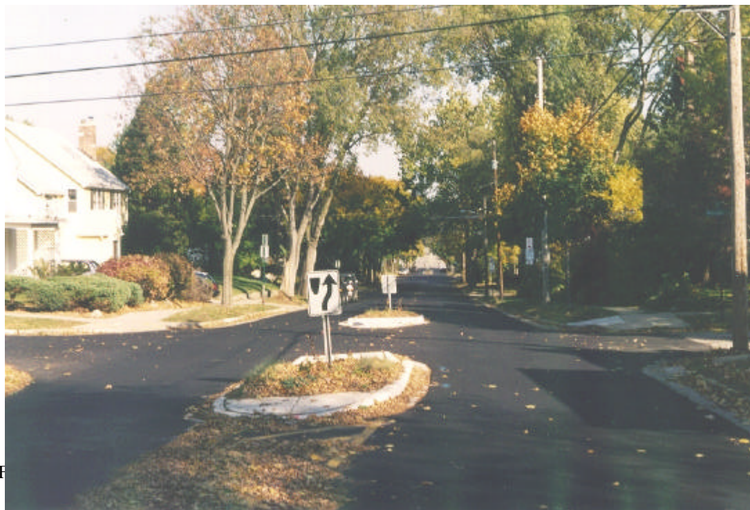
Figure 11. Local residential street pedestrian refuge islands (Islands on Thompson Drive will differ).
