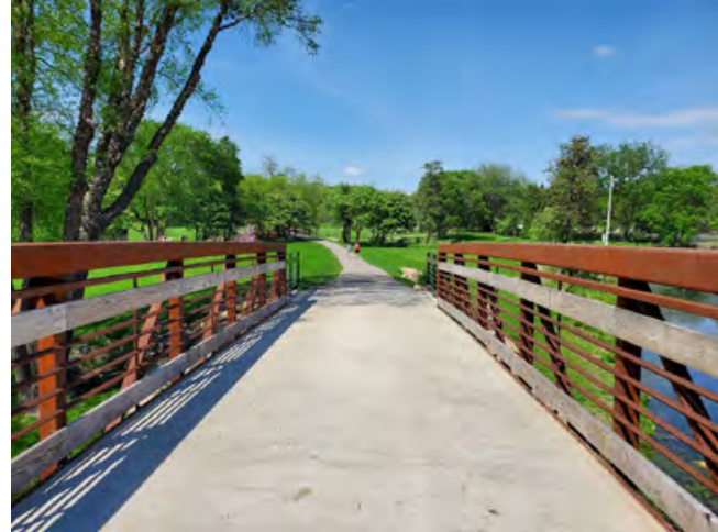
Figure 5.56. Bridge Concrete Surfacing
