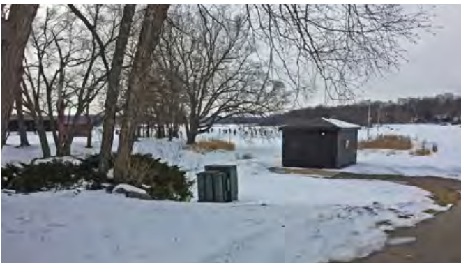
Figure 5.11. Pump House in Winter
