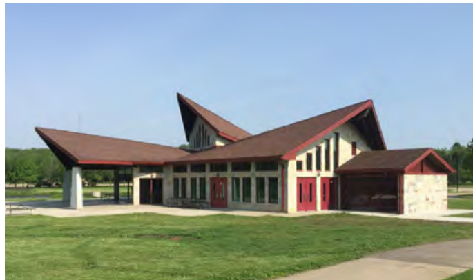
Figure 6.5. Elver Park Shelter
