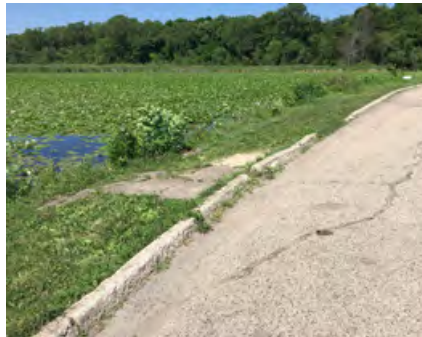
Figure 5.32. Drain Trench to Lake
