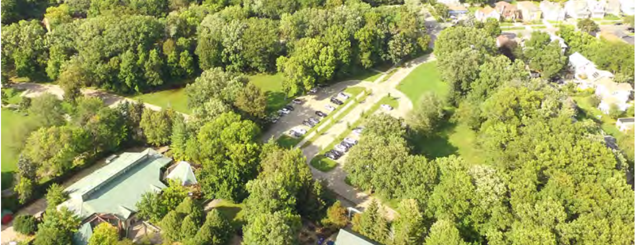
Figure 7.10. Existing North Parking Lot
