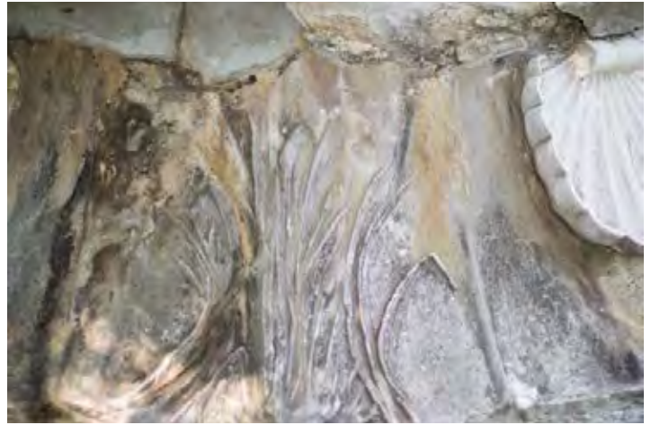
Figure 53: View of degraded material at cattail motif
