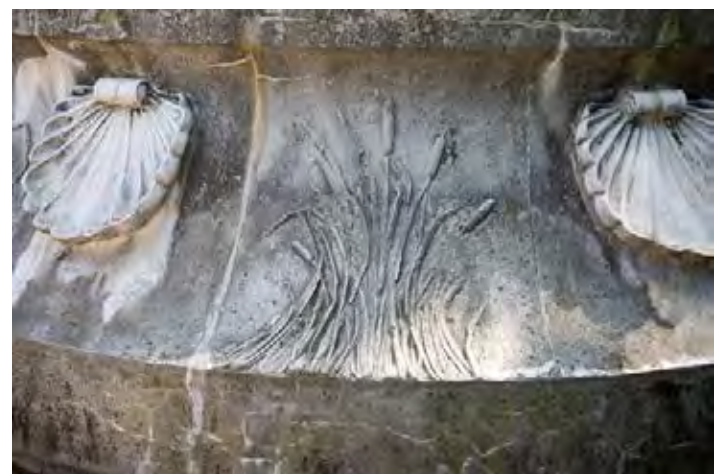
Figure 34: Relatively intact stone to concrete transition
