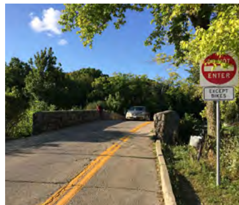
Figure 5.53. Stonework of Bridge
