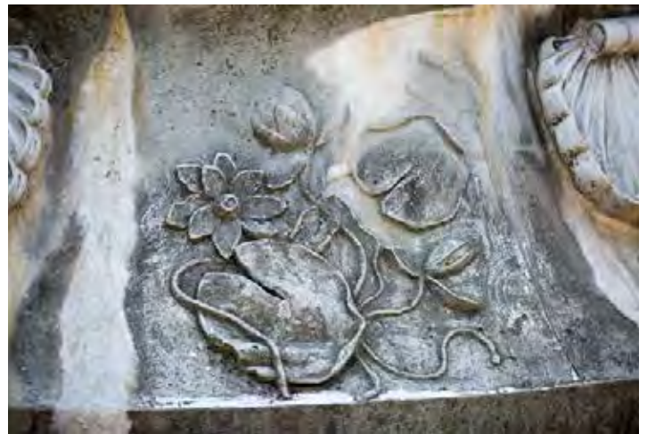
Figure 36: View of intricate detail at base, mineral deposits at trailing water
