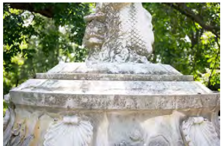
Figure 19: Relatively intact base/pedestal transition
