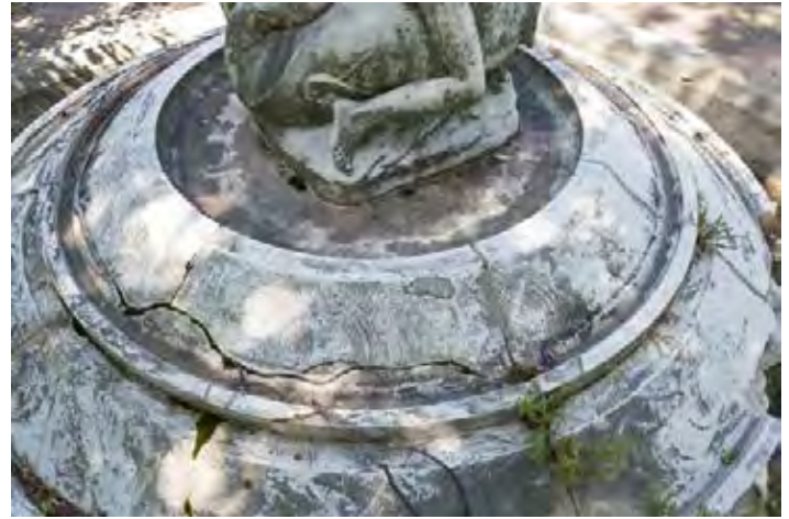
Figure 5: Upper view of pedestal and base - note damage to pedestal has been repaired and appears to have stabilized
