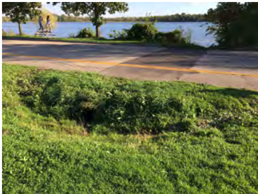
Figure 5.34. Storm Drain at VPD
