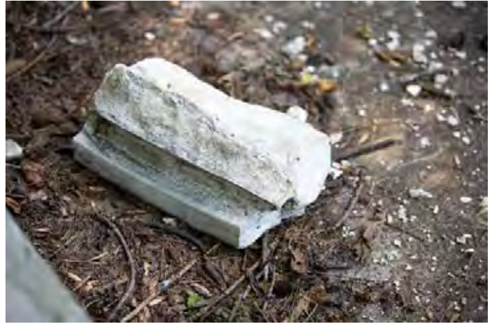
Figure 23: Broken piece on the site
