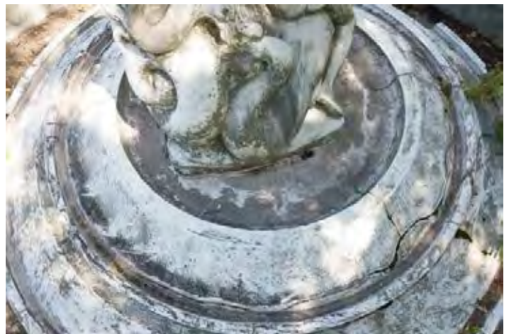
Figure 7: Upper view of pedestal and base - note damage to pedestal has been repaired and appears to have stabilized
