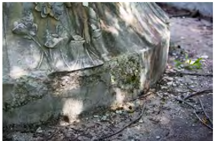
Figure 31: Stone to concrete transition
