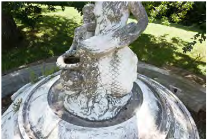
Figure 12: View of dolphin figure - note the apparent loss of detail from organic buildup
