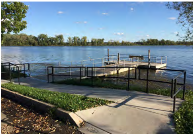
Figure 5.137. ADA Pier on Lake Wingra at Vilas Park
