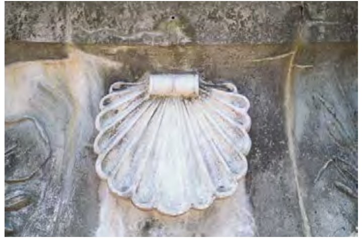
Figure 47: View of weep holes, cracked limestone mineral deposits and trailing water
