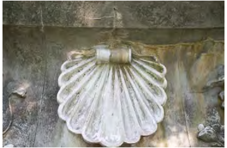
Figure 50: View of weep holes, cracked limestone mineral deposits and trailing water
