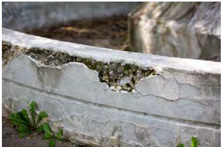
Figure 24: Coarse ring aggregate concrete at lower perimeter
