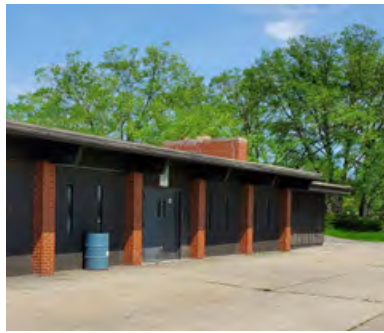
Figure 5.2. Shelter Tuck Pointing
