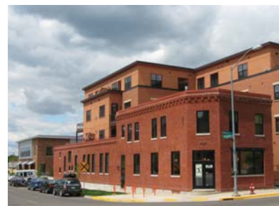
B2. Variation in roof lines
