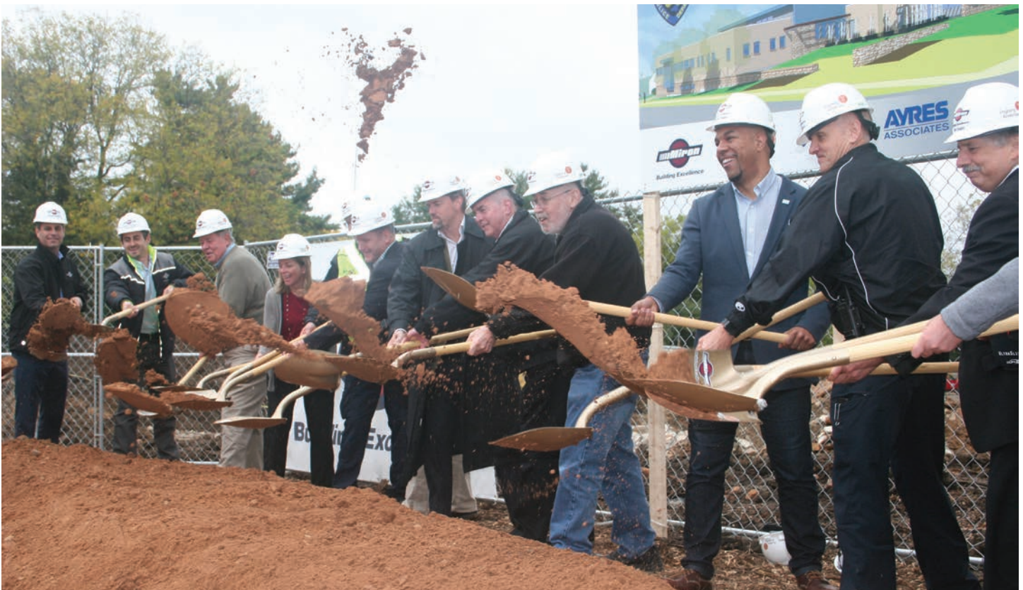
Midtown Station Groundbreaking.
