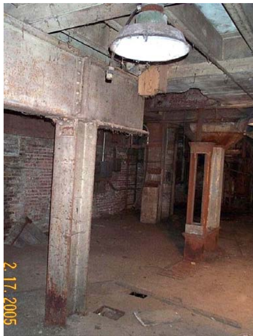
Figure 33, original cup conveyor equipment
