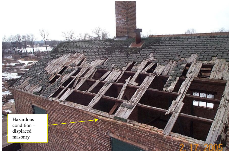
Figure 32, displaced masonry at boiler building
