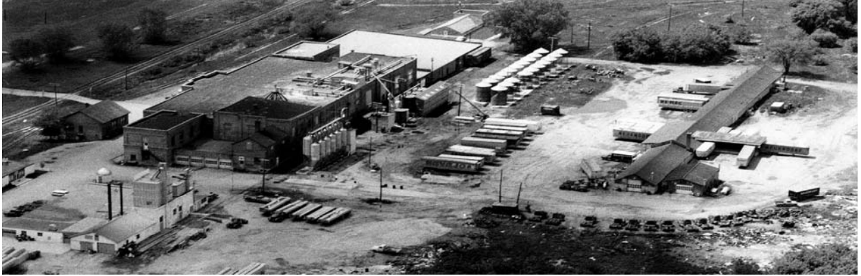
Figure 22: Detail of an undated aerial view circa the early 1960s showing roof transitions and the small Prater Package Feed Plant on the roof of Building 7. Also note the numerous tanks that have been installed at the rear of the building subsequent to the earlier photo series.
