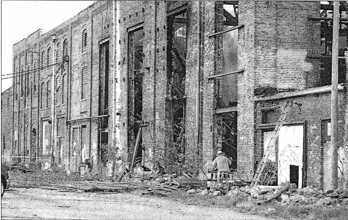
Figure 29, May, 2001 Photograph of the fire-damaged rear elevation of the main building. Note the uniform cornice line despite very different fenestration patterns at each section of the building. Photo credit: John Maniaci/Wisconsin State Journal.
