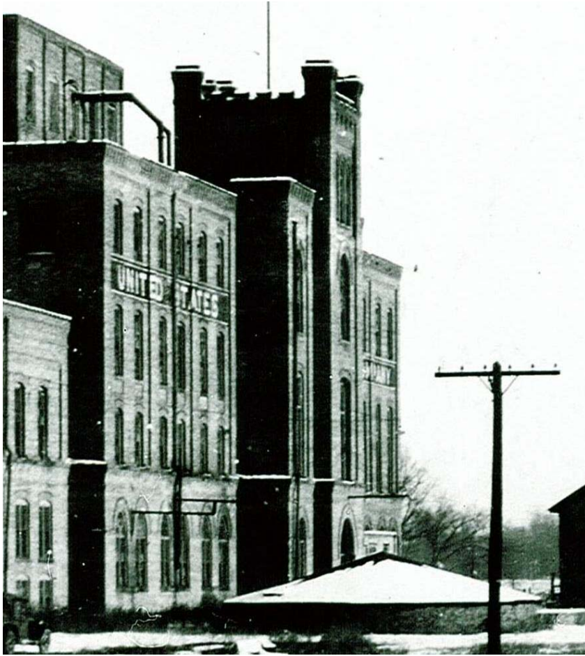
Figure 6: Detail of the south elevation of the main building. The low round building in the foreground is noted as a molasses tank on the 1908 Sanborn map. Immediately above the peak of the roof of the tank, a light-colored enclosure is visible east of the main entrance of the processing plant.
