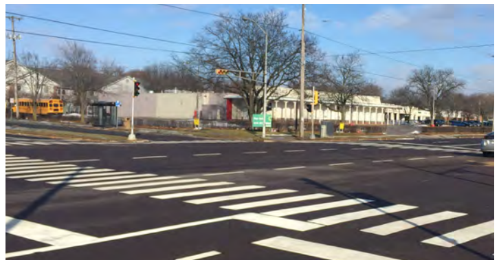
Example of a continental crosswalk on Cottage Grove Road.
