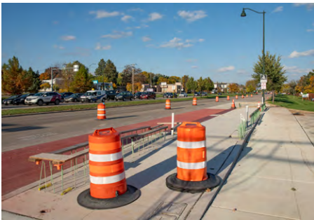
East Washington Avenue - construction of BRT station
