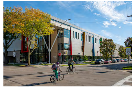
The Madison Youth Arts building on East Mifflin Street exemplifies effective use of facade articulation, offering diverse design elements that enhance visual appeal and create an inviting atmosphere for pedestrians.
