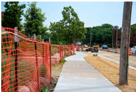
Small physical improvements example - sidewalk repair
