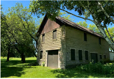
Amund Reindahl's barn, located in Reindahl park
