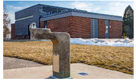
Madison Water Utility's Well 15
