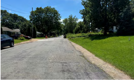
Lack of sidewalks near Hawthorne Elementary School
