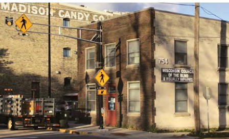
Rectangular rapid flashing beacon (RRFB)
