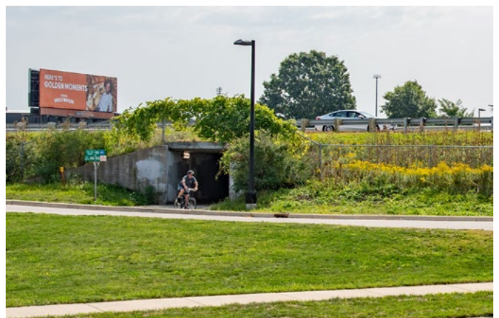
The Struck Street underpass of the Beltline is an important connection for pedestrians and bicyclists, but is in need of upgrades.
