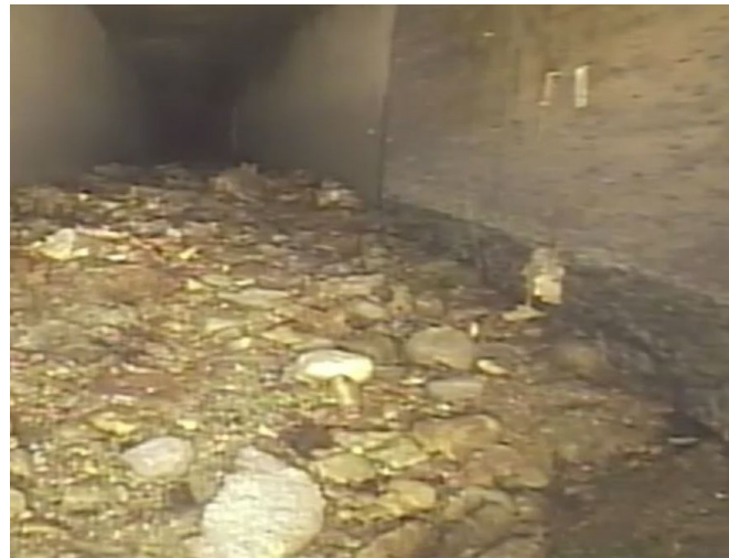
PATCH W/PLYWOOD FORM IN PLACE, GRAVEL ACCUMULATION
