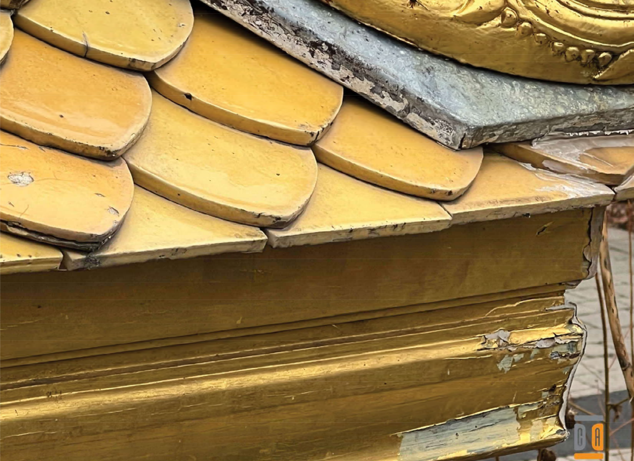
21. Repair attempts at base of hip ridge - Priority 1
