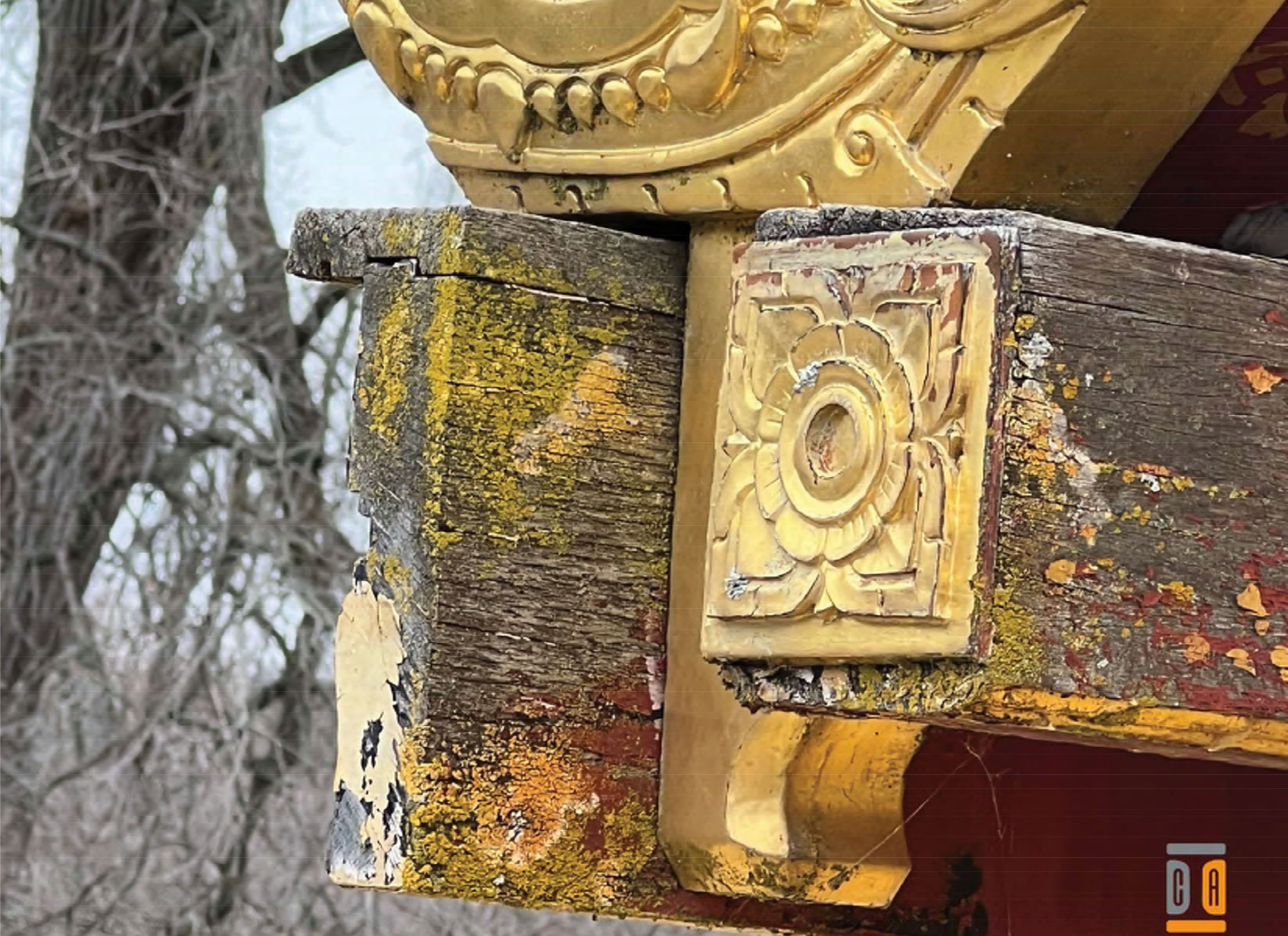
41. Repair attempts at base of hip ridge - Priority 2
