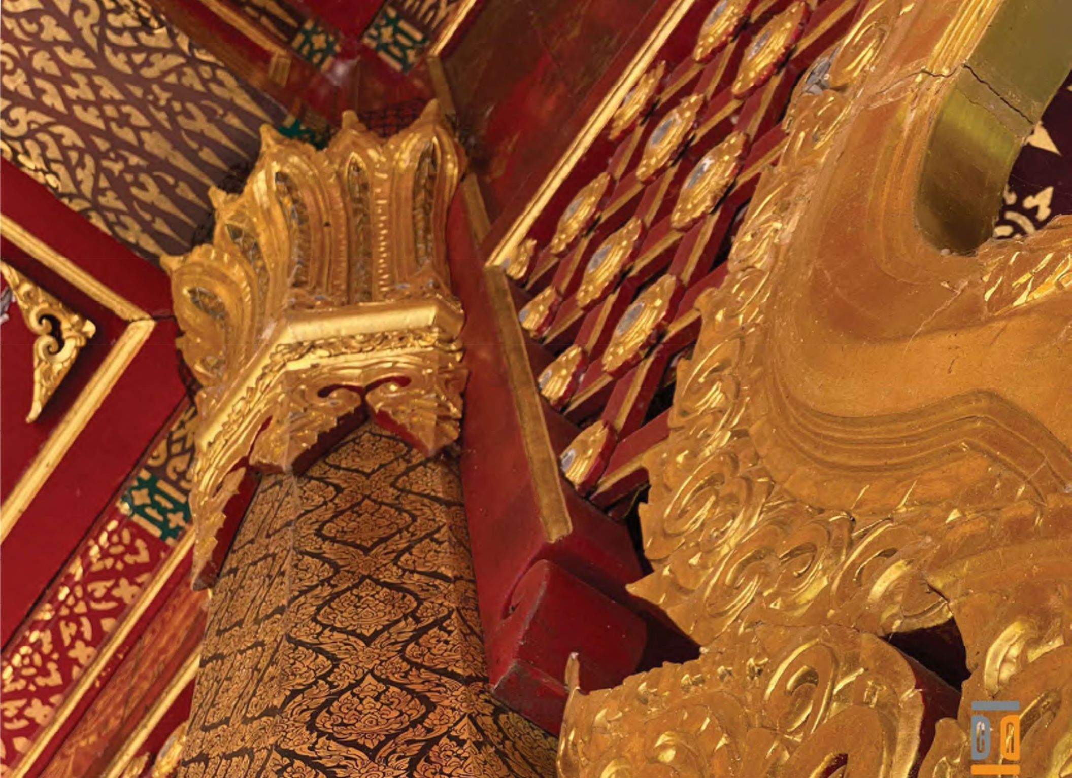
47. Interior Condition of column capital - Priority 2
