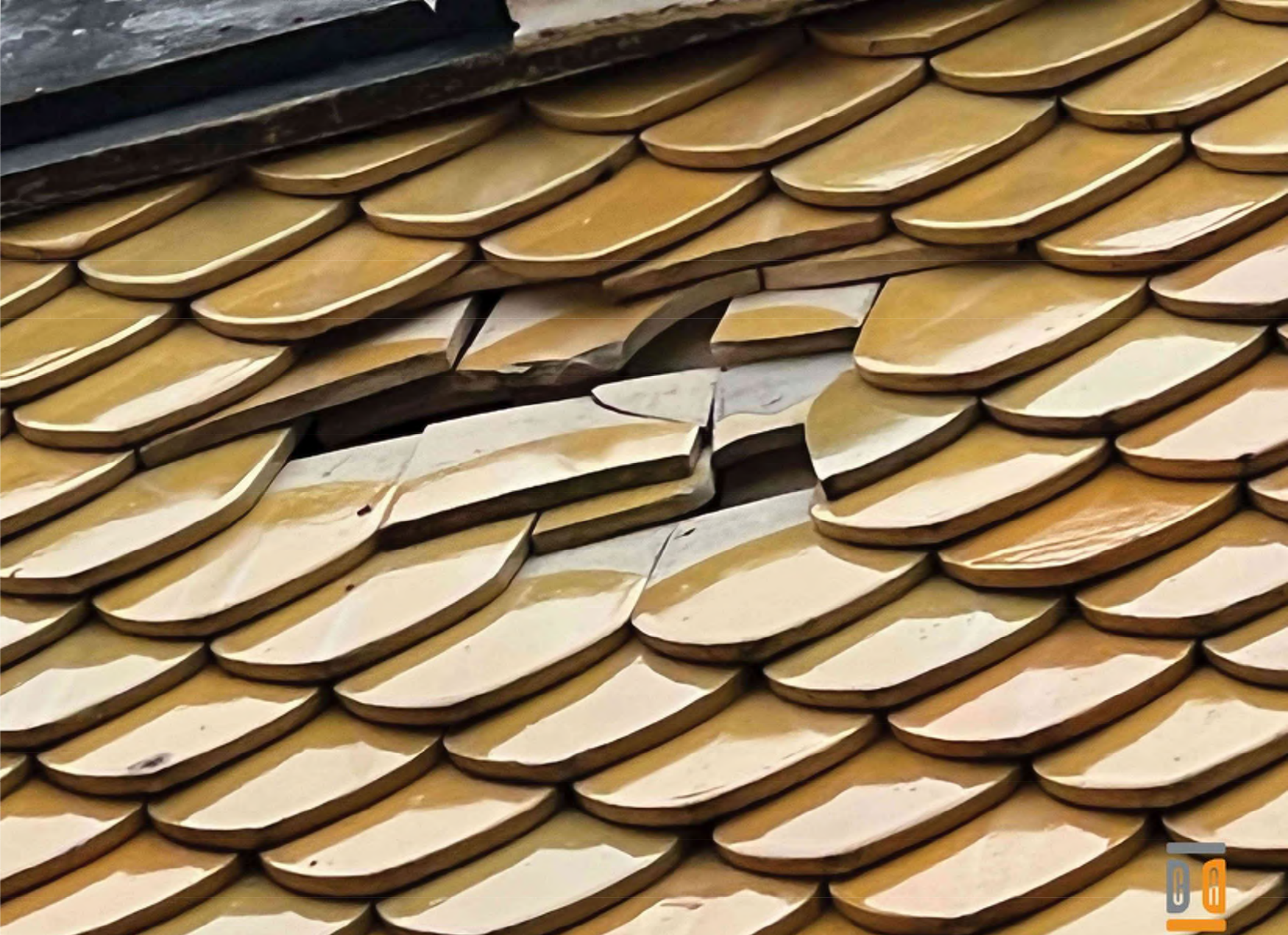
14. View of fractured tile – from impact or concentrated point load (assumed) - Priority 1
