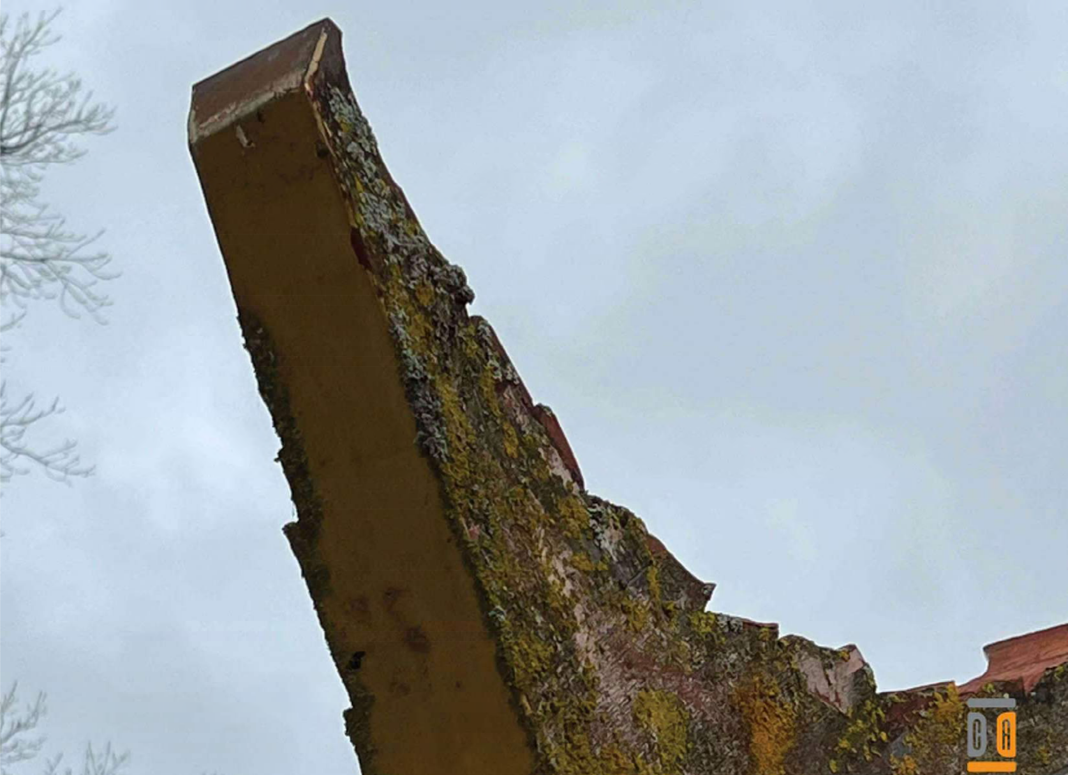
31. Batter boards at rake close-up leads are gone, finishes failed, biological growth, wood is sound - Priority 1
