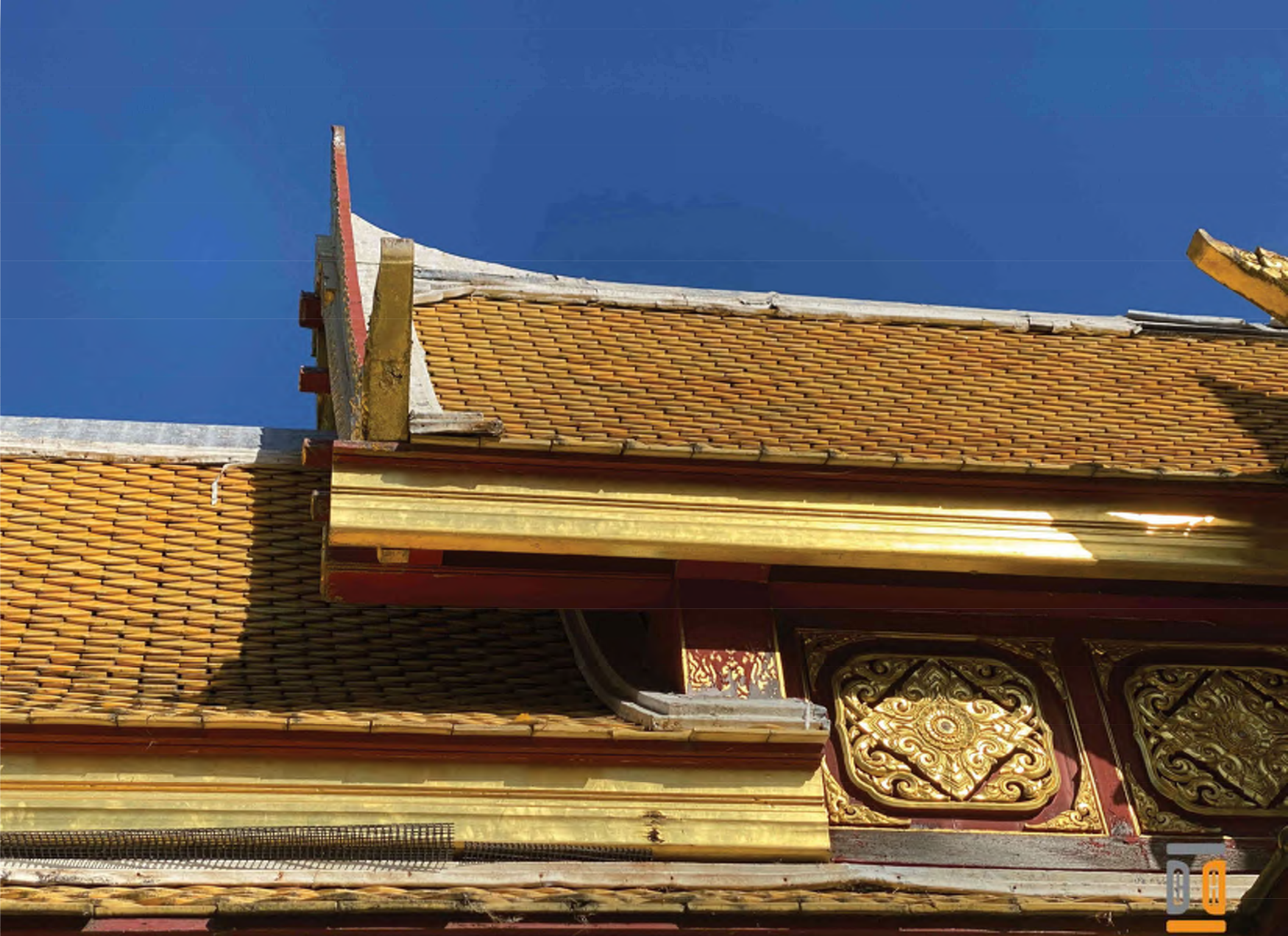
35. West view of upper roof condition - Priority 1
