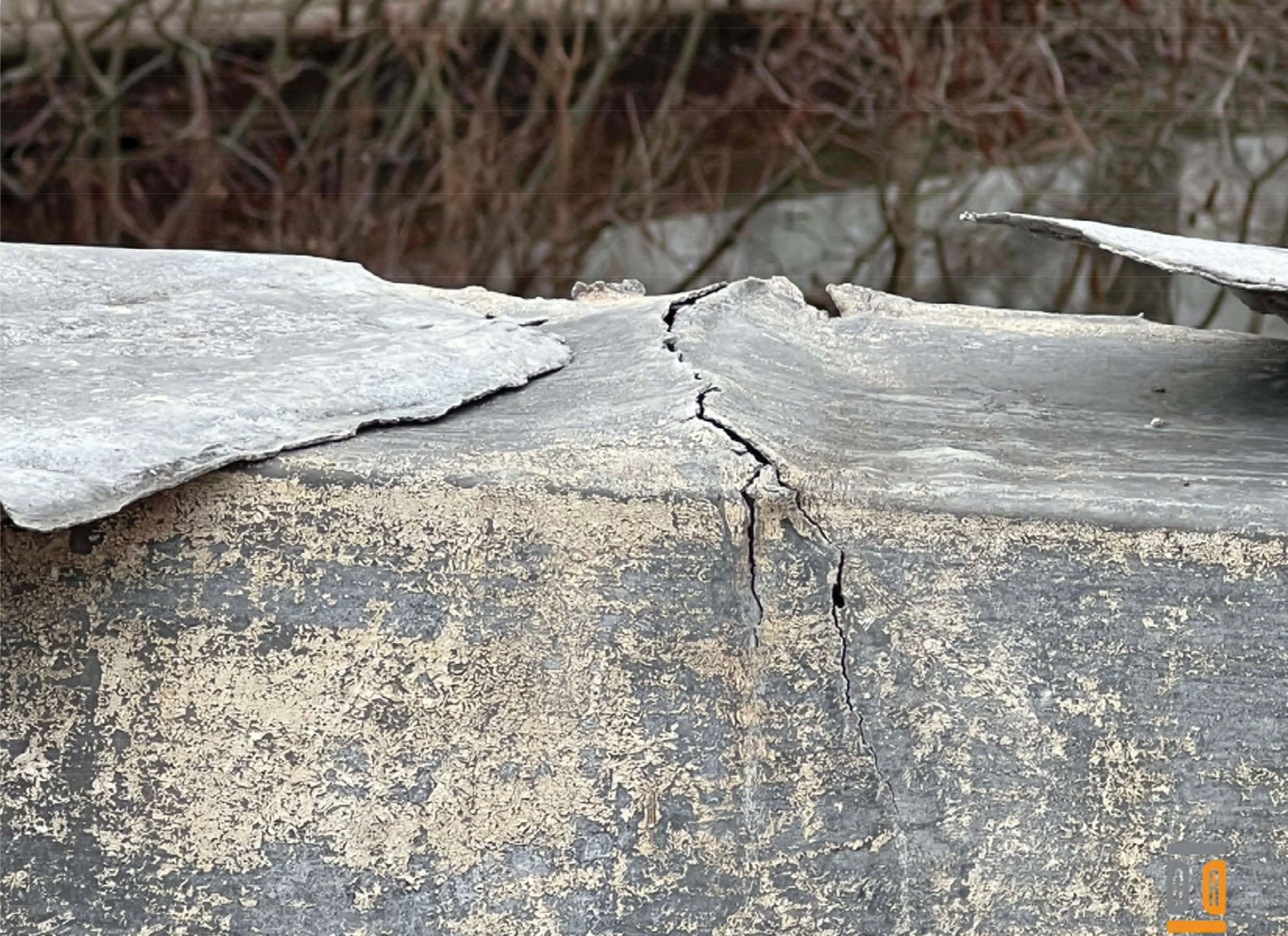
32. Degraded and fractured lead fasteners failure has led to cyclic fatigue and critical failure - Priority 1
