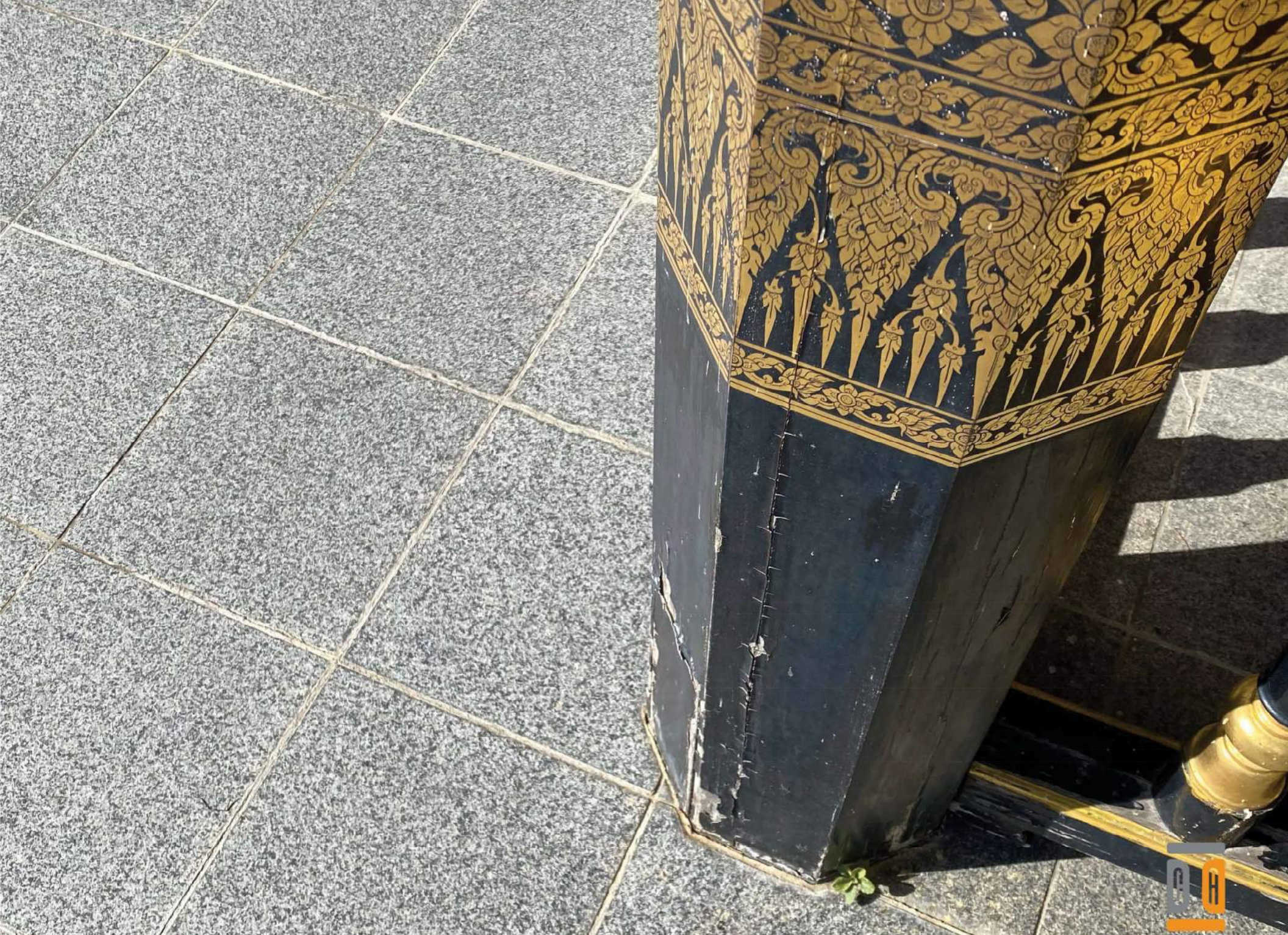
52. Column Base Condition with buckling wood seams and some dry rot - Priority 2
