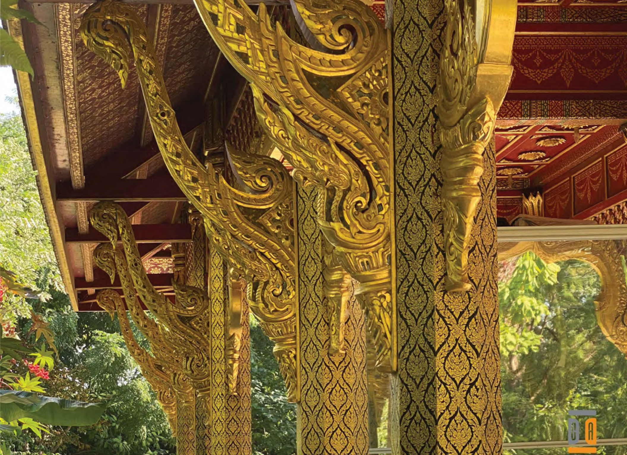
48. Exterior Condition of column capital - Priority 3
