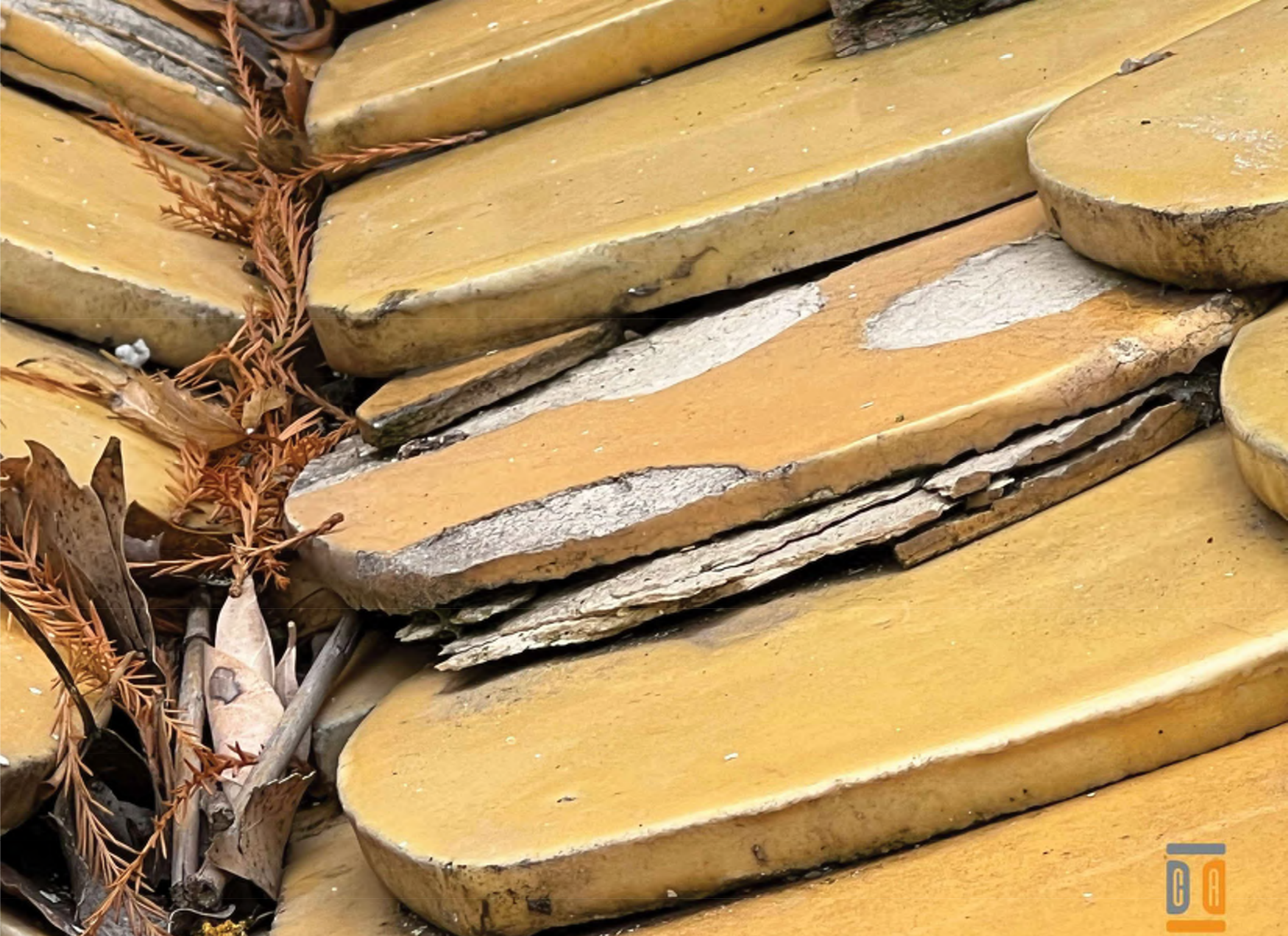
19. Close up of tile degradation at valley identified in images - Priority 1
