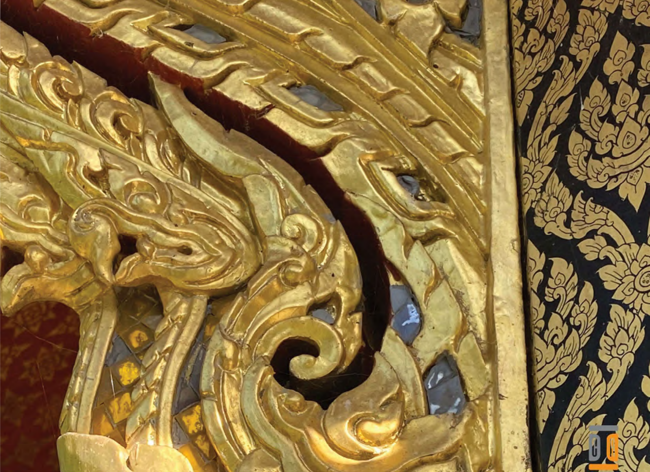
50. Exterior Condition of column capital - Priority 3
