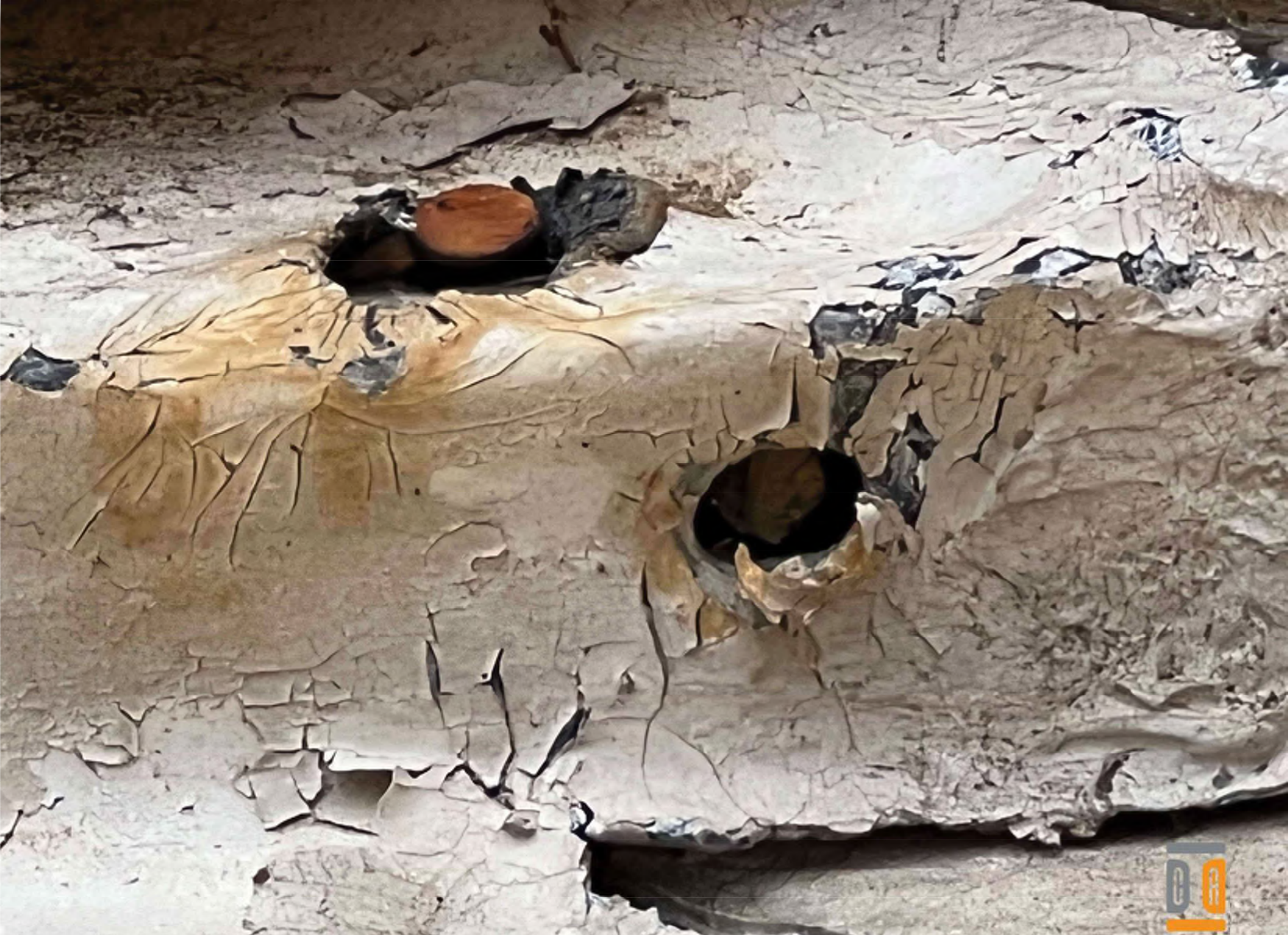
26. Failure as lead – galvanic cell oxidation failure - Priority 1
