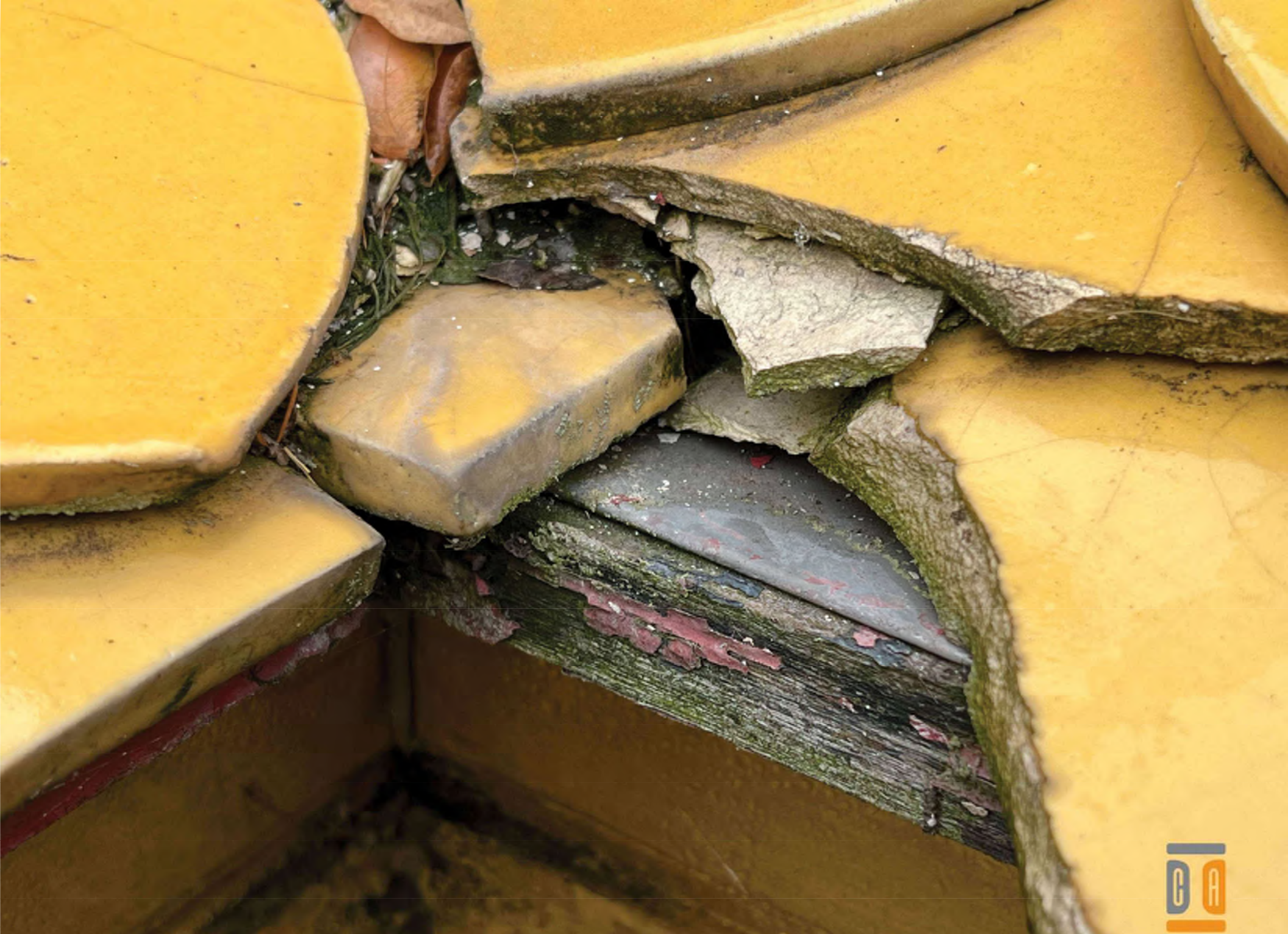
20. Close-up of valley termination at location referenced in images - Priority 1
