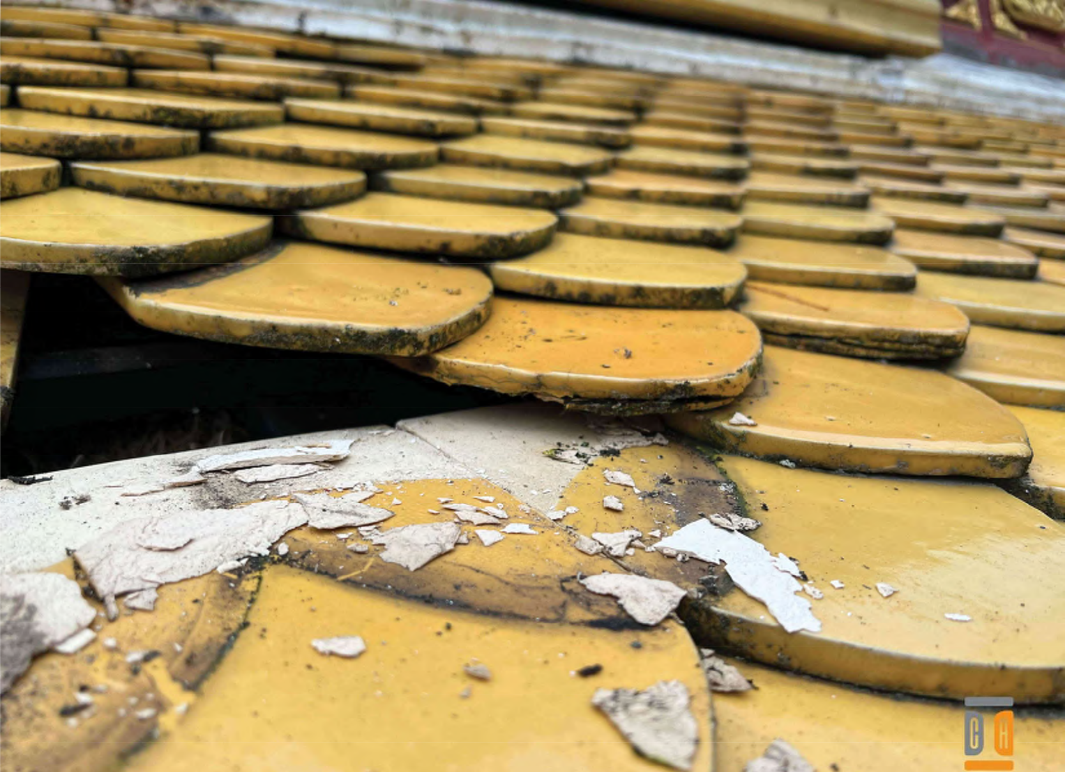
10. Removed tile location relating to #8 (above) - Priority 1
