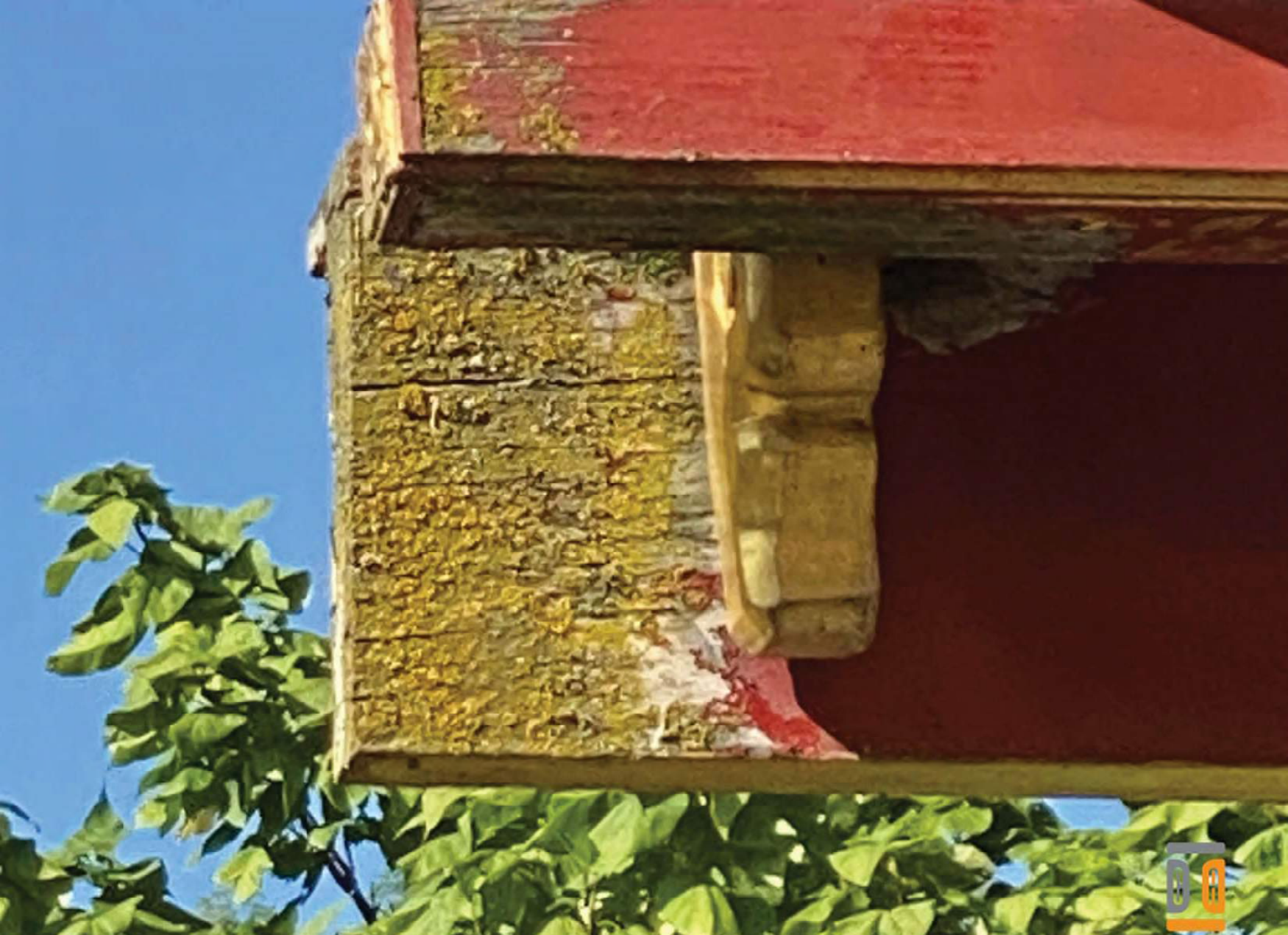
42. Representative image of degradation observed to finishes and wood substrate - Priority 2
