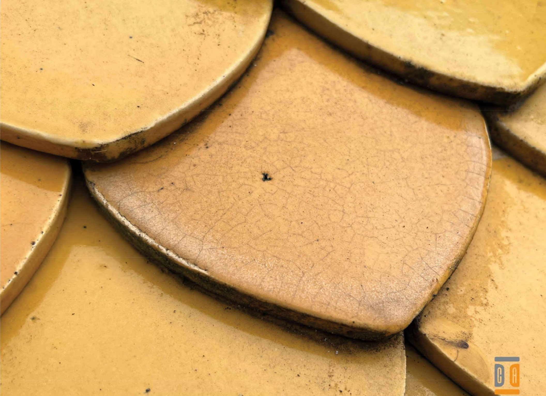
15. Fractured ceramic glaze – eventual water infiltration - Priority 1
