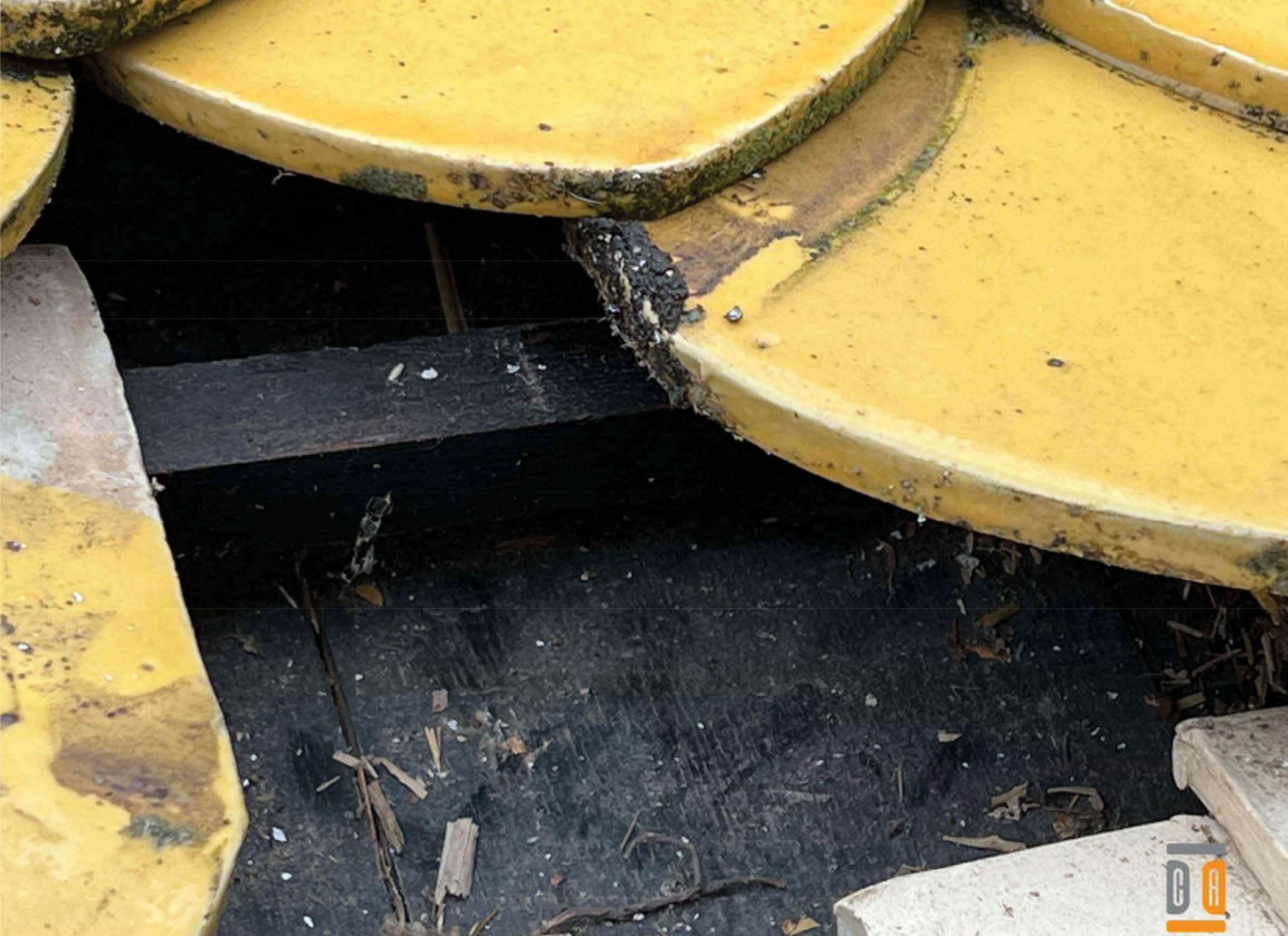
7. Roof Substructure without underlayment. Asphaltic (bituminous) coating on wood - Priority 2
