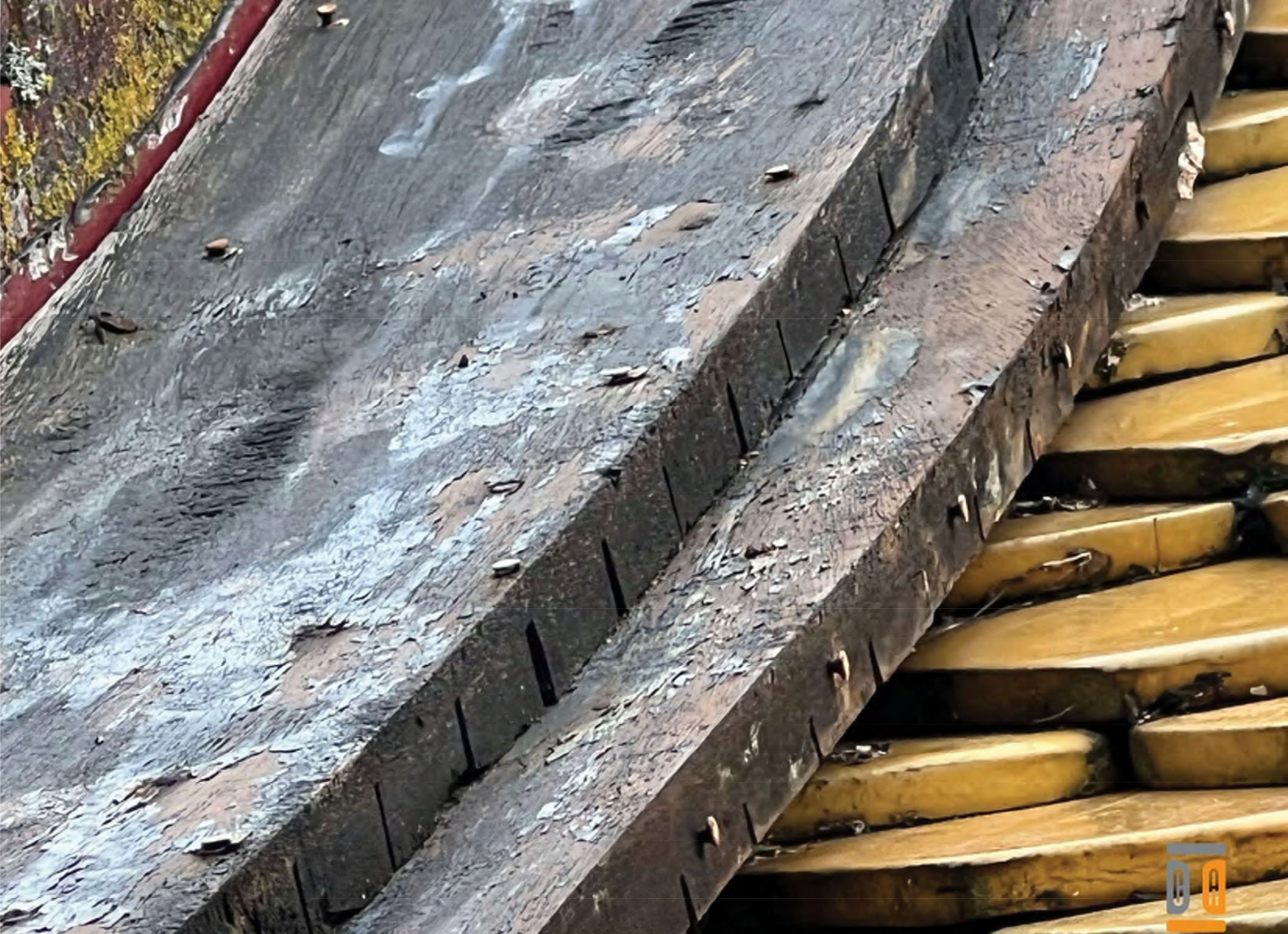
29. Batter boards at rake close-up, leads are gone, finishes failed wood is sound, note kerfs in sweat batter board and note failed coating - Priority 1
