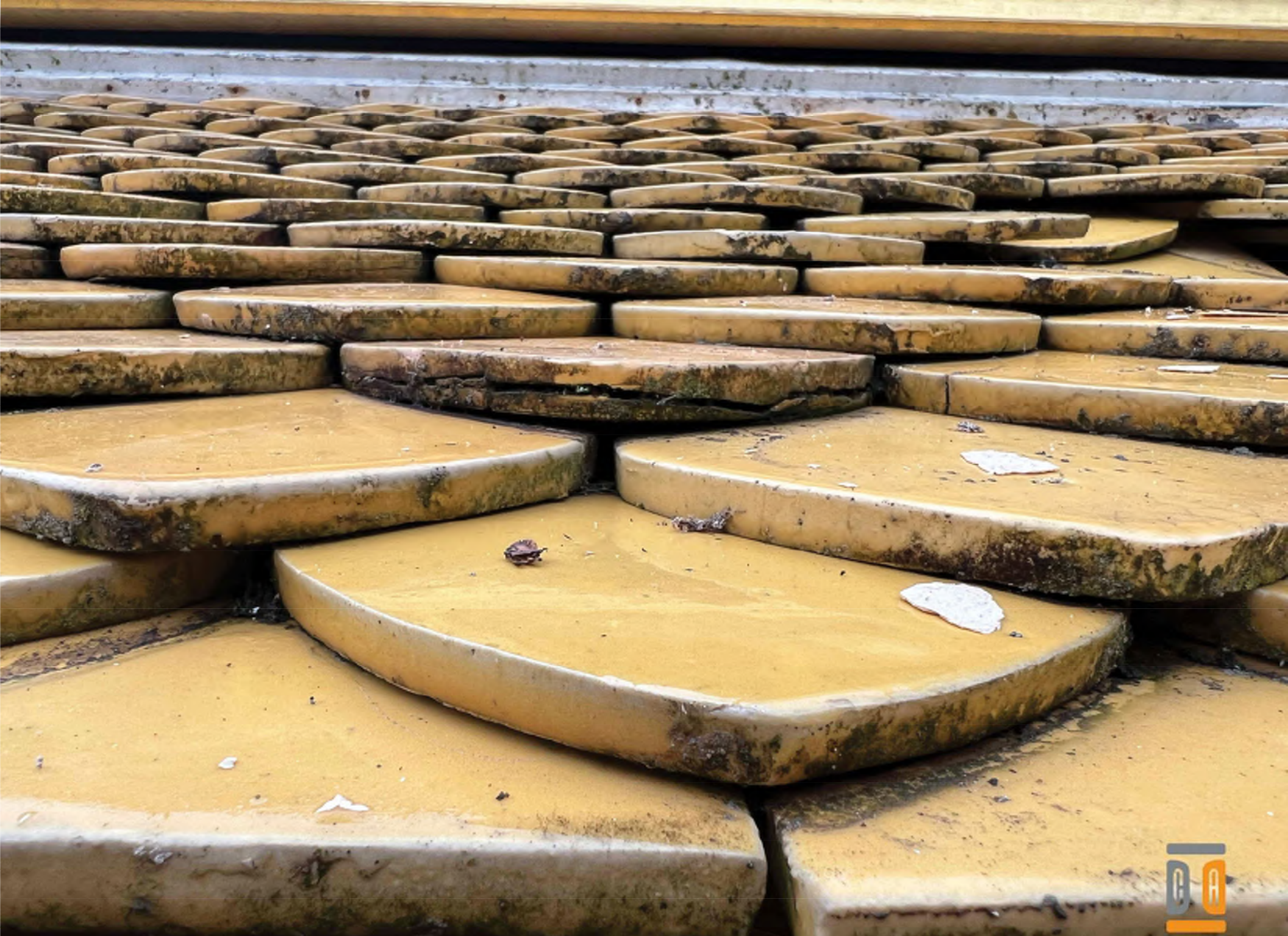
5. Tile debris at top of down-slope - Priority 1
