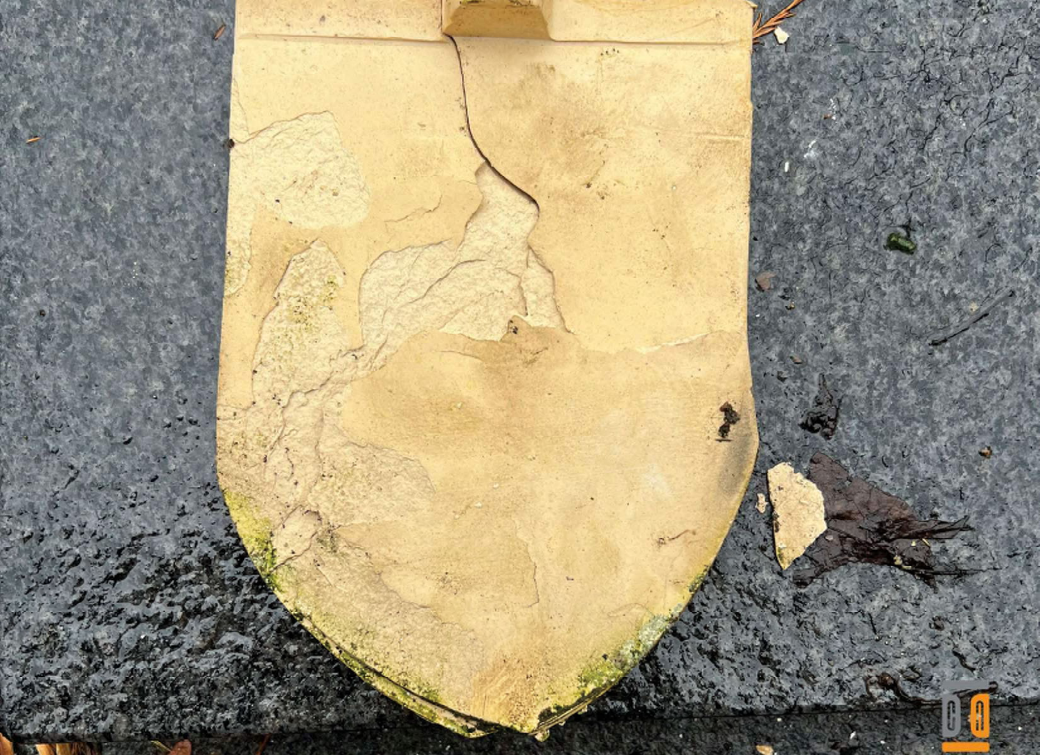
9. Reconstructed tile - Typical condition of water-infiltration damage - Priority 1
