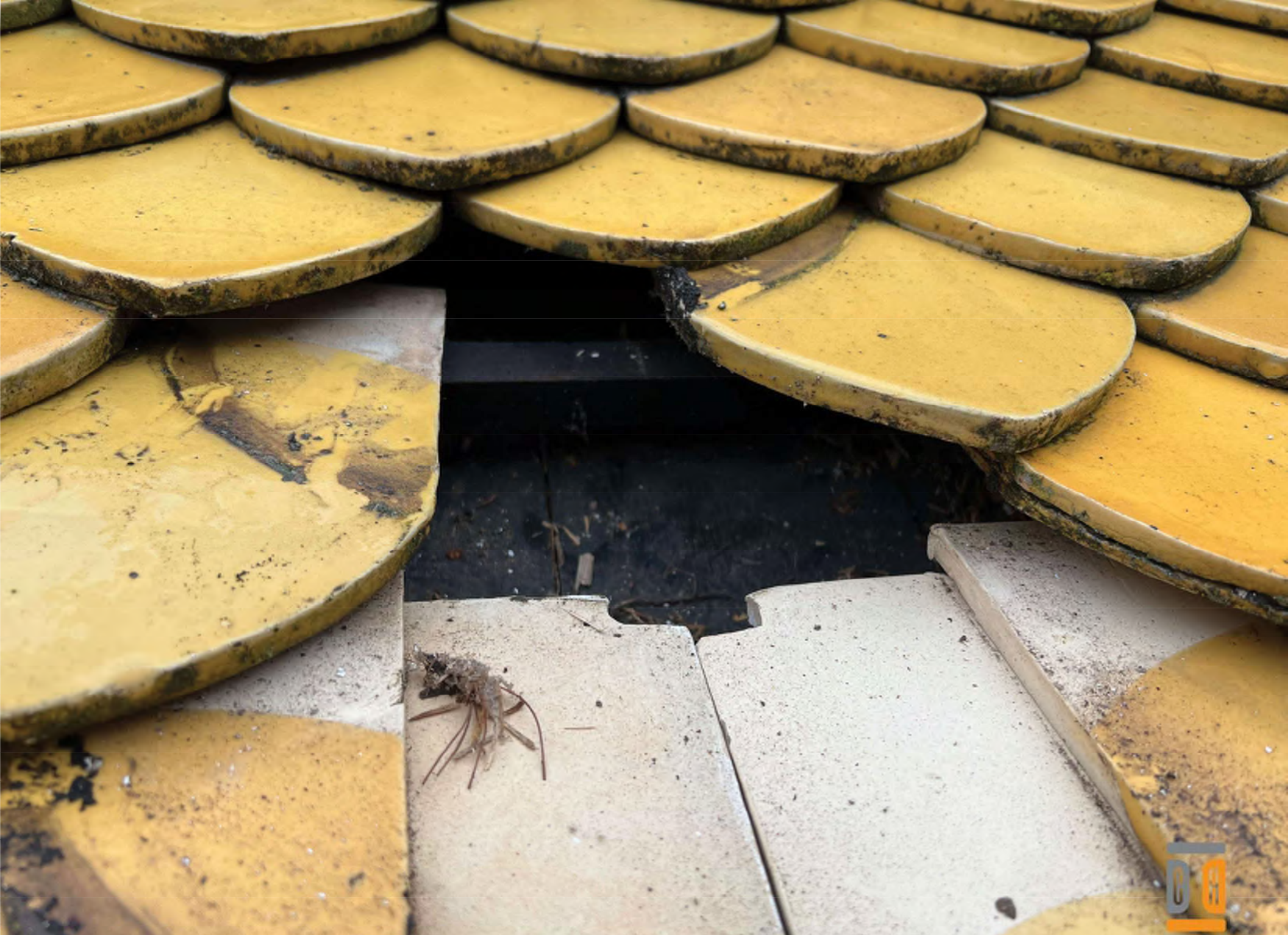
6. Failure mode, laminar failure, expansive clay soluble salt capillary action water crystallization/expansion - Priority 1
