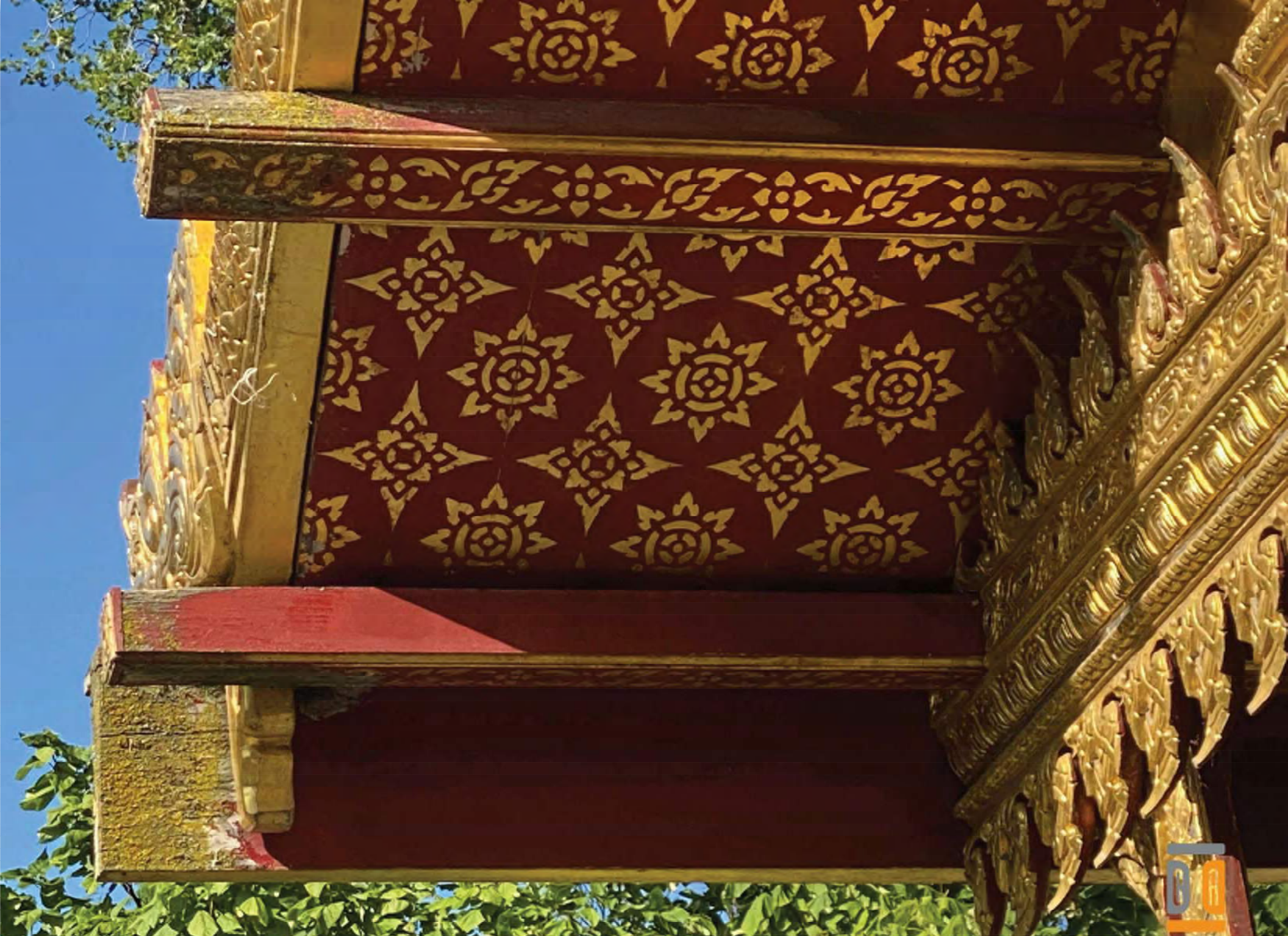
39. View of soffit and wood components showing dry-rotted wood and paint failures - Priority 2
