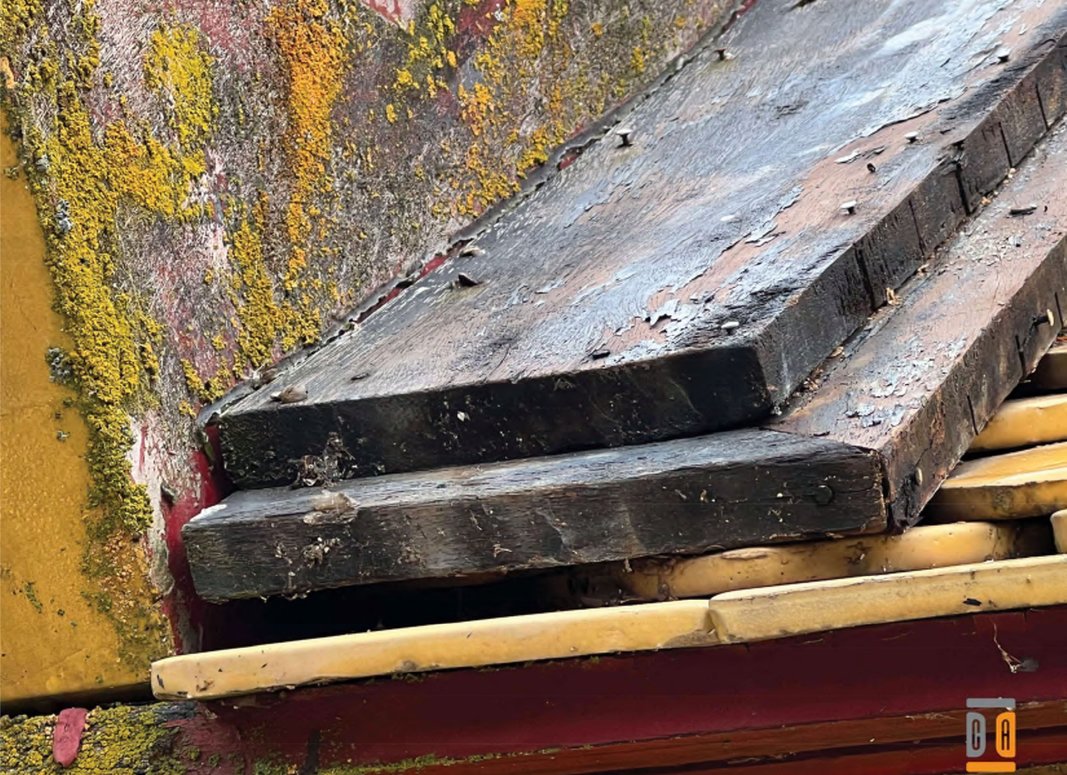
28. Batten boards at rake close-up, leads are gone, finishes failed wood is sound, and biological growth - Priority 1
