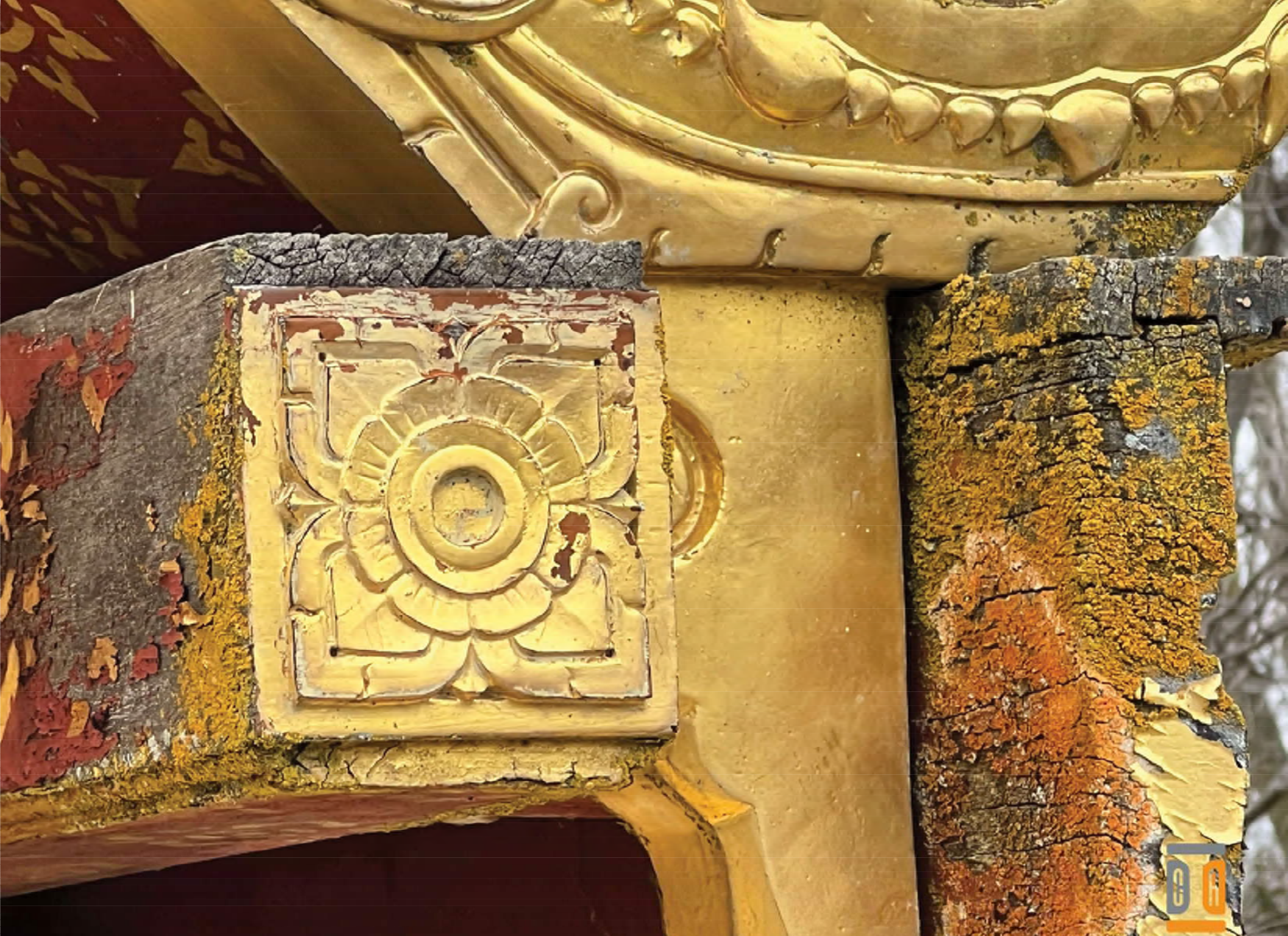
40. Representative image of degradation observed to finishes and wood substrate - Priority 2
