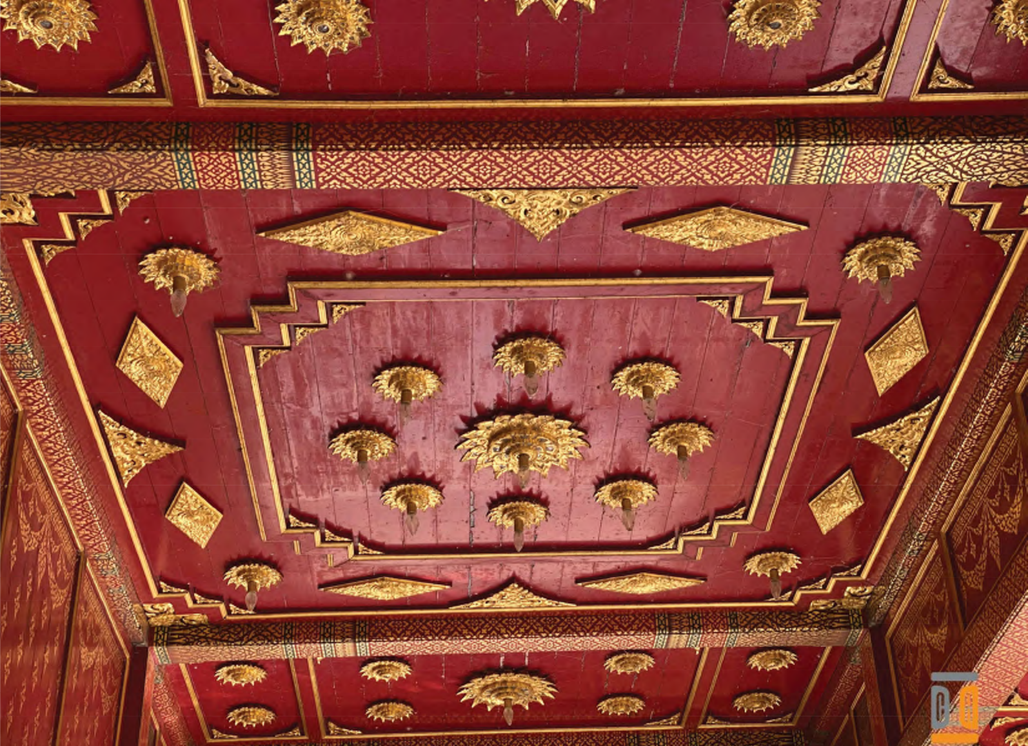
44. Interior Ceiling condition with buckling edges and paint failure - Priority 2
