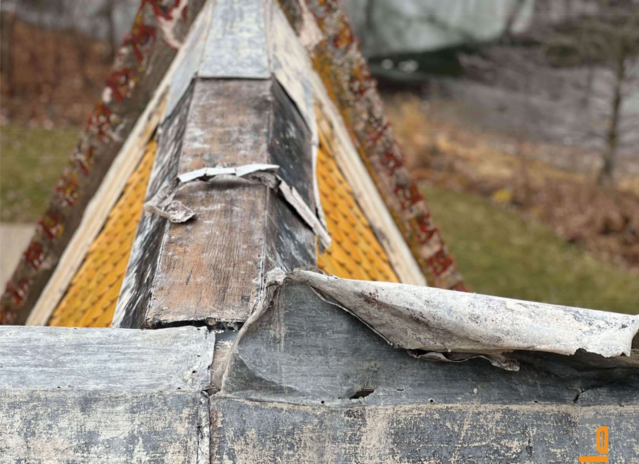
33. Lead failure at intersecting ridges - Priority 1
