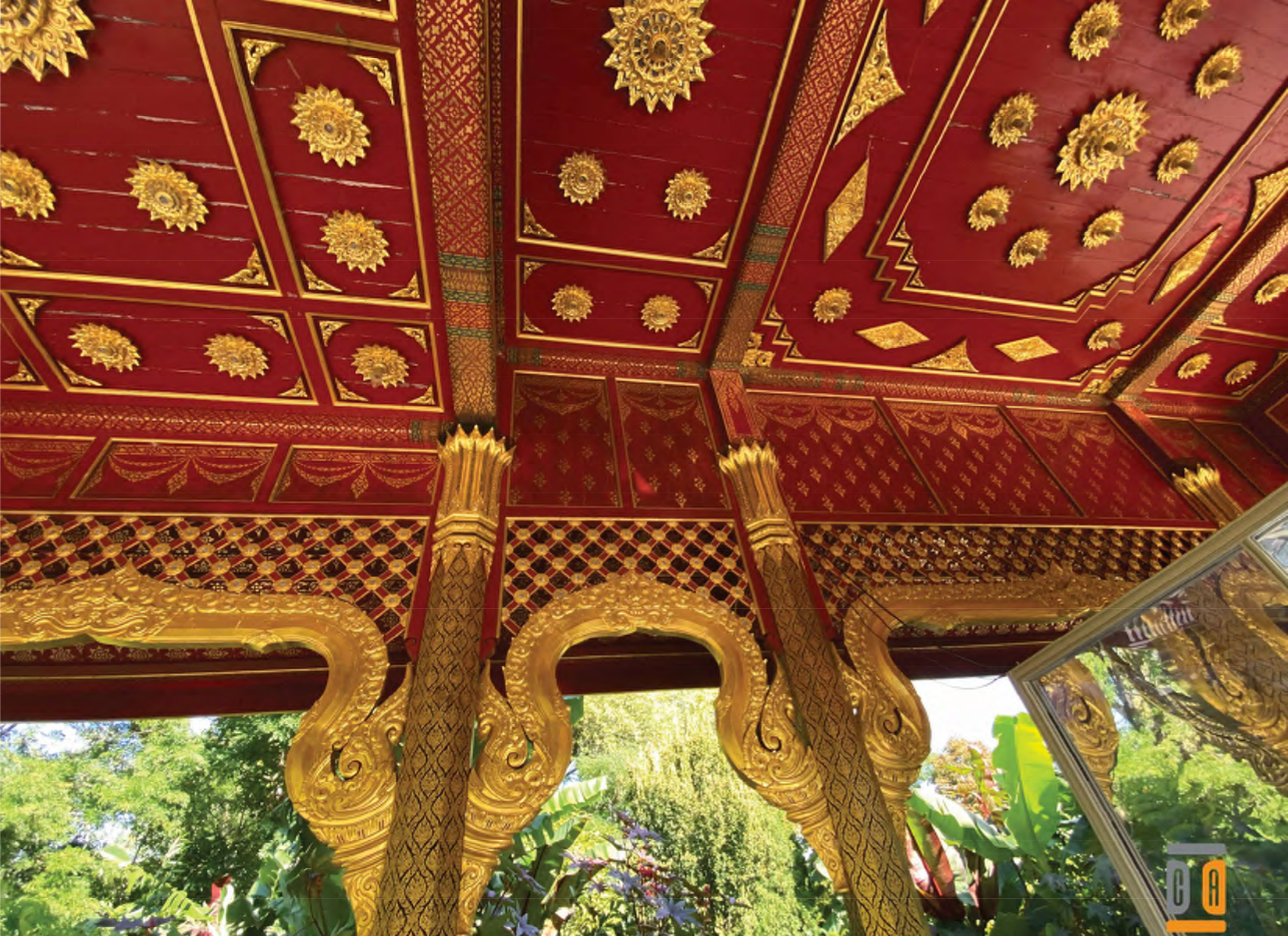
45. Interior Ceiling condition with buckling edges and paint failure - Priority 2
