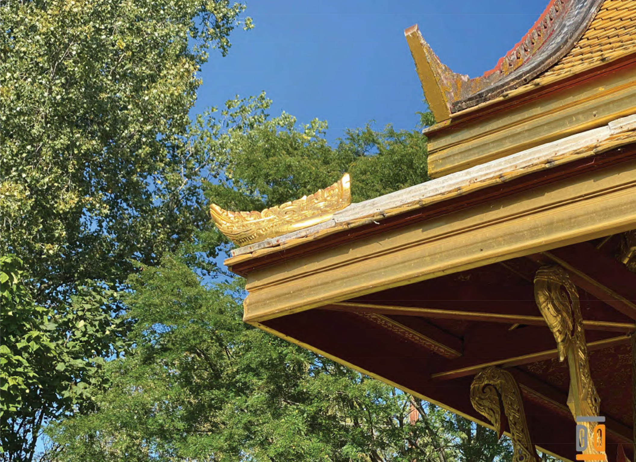
37. Corner view of North Gable end - Priority 2
