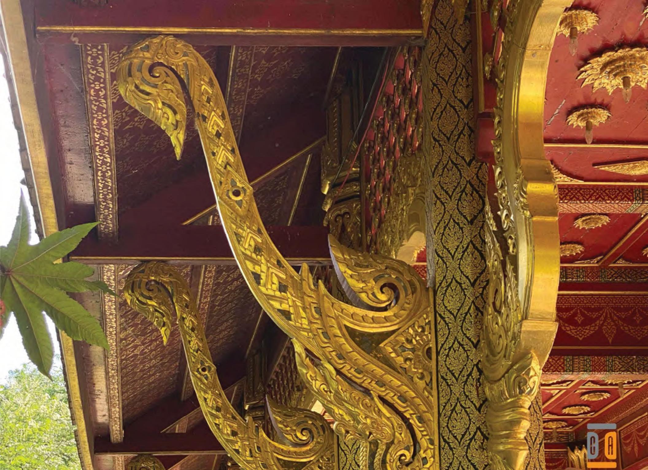
49. Exterior Condition of column capital - Priority 3
