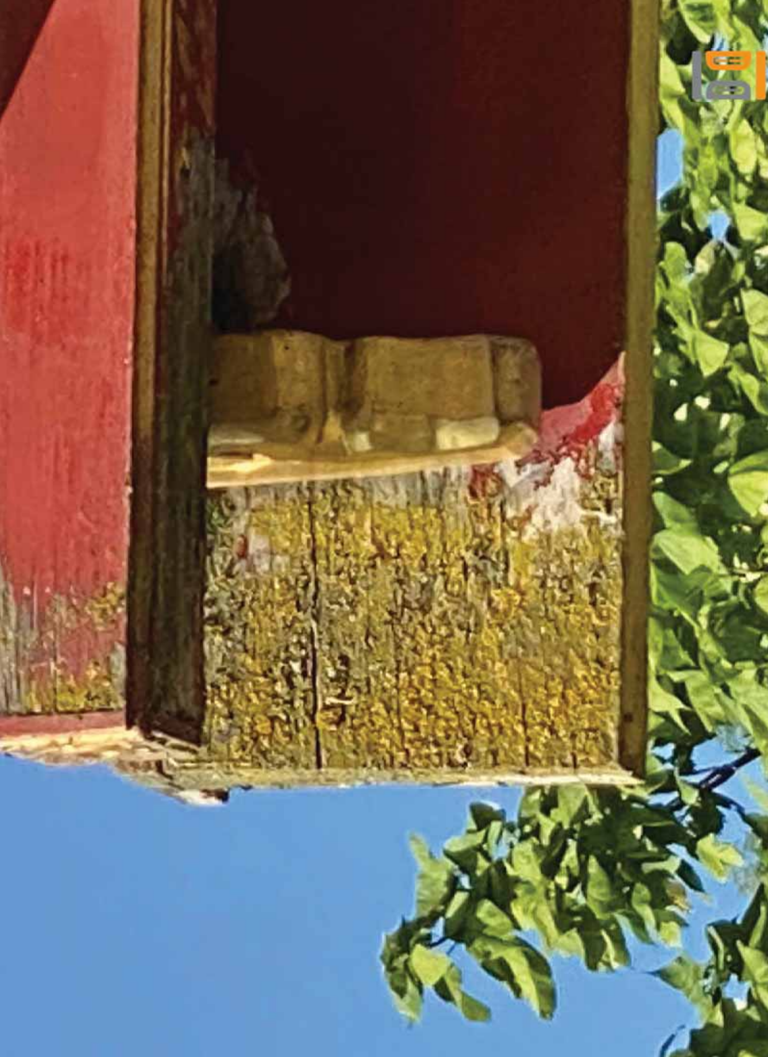
42. Representative image of degradation observed to finishes and wood substrate - Priority 2
