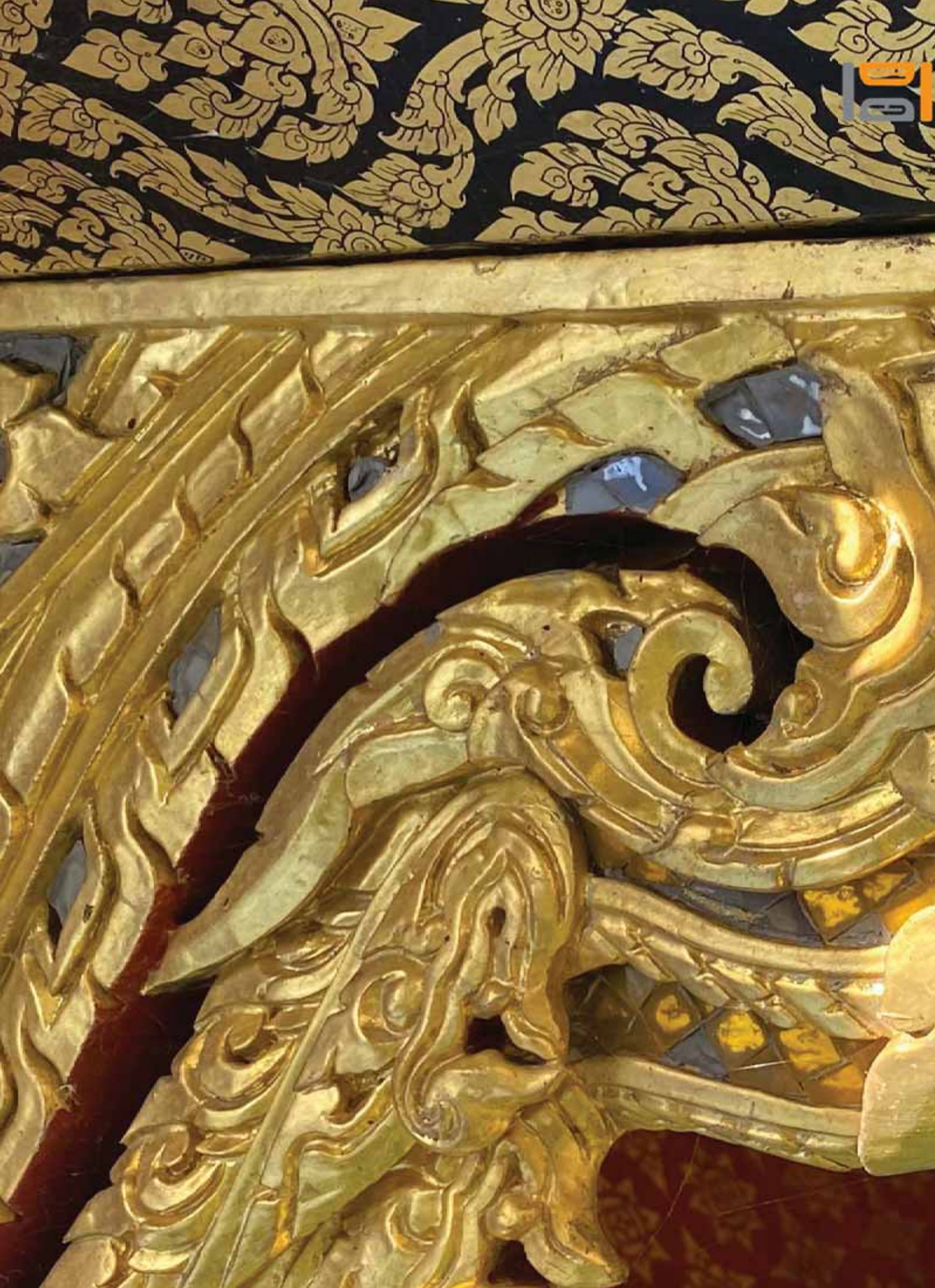
50. Exterior Condition of column capital - Priority 3
