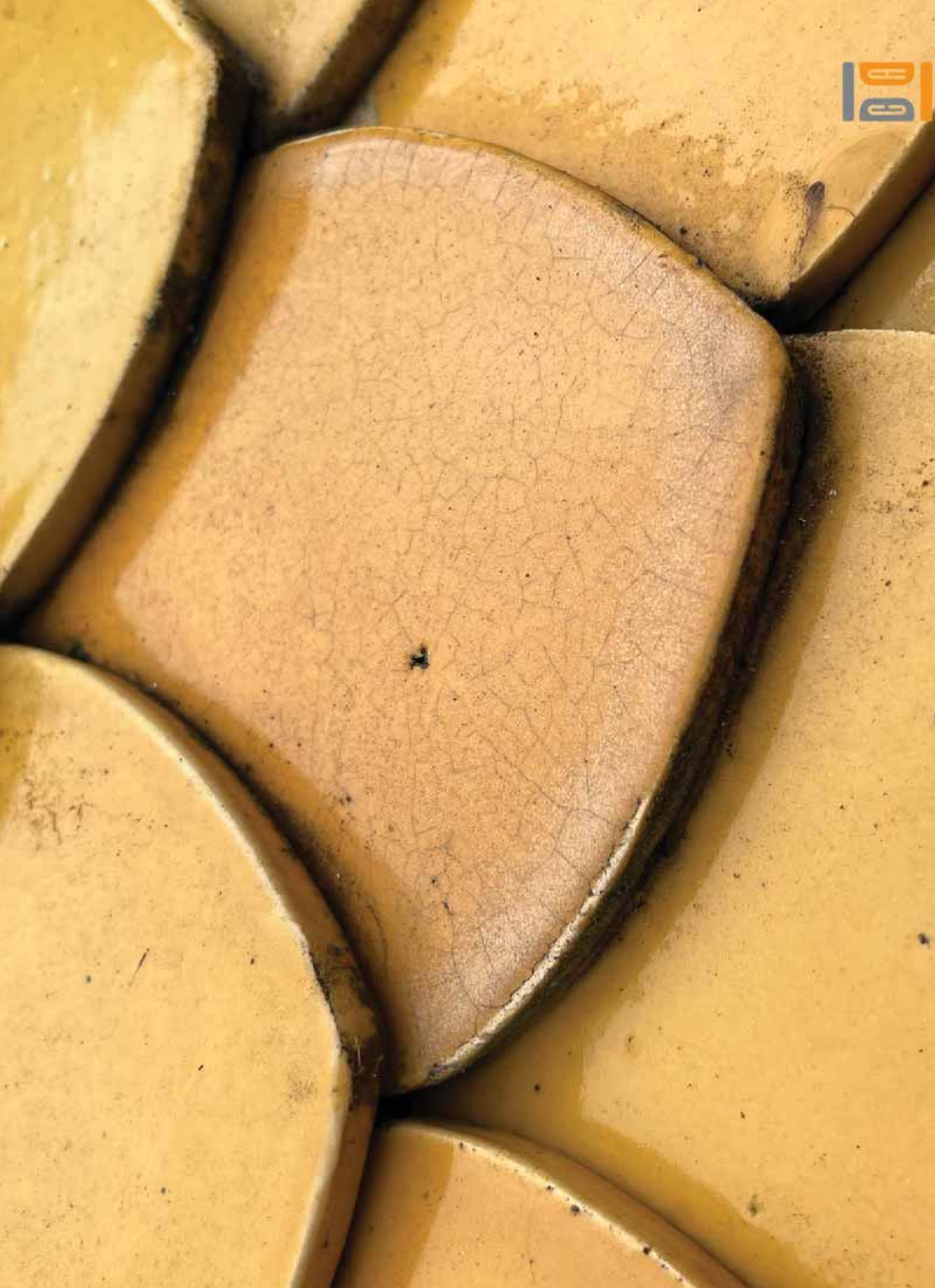
15. Fractured ceramic glaze – eventual water infiltration - Priority 1
