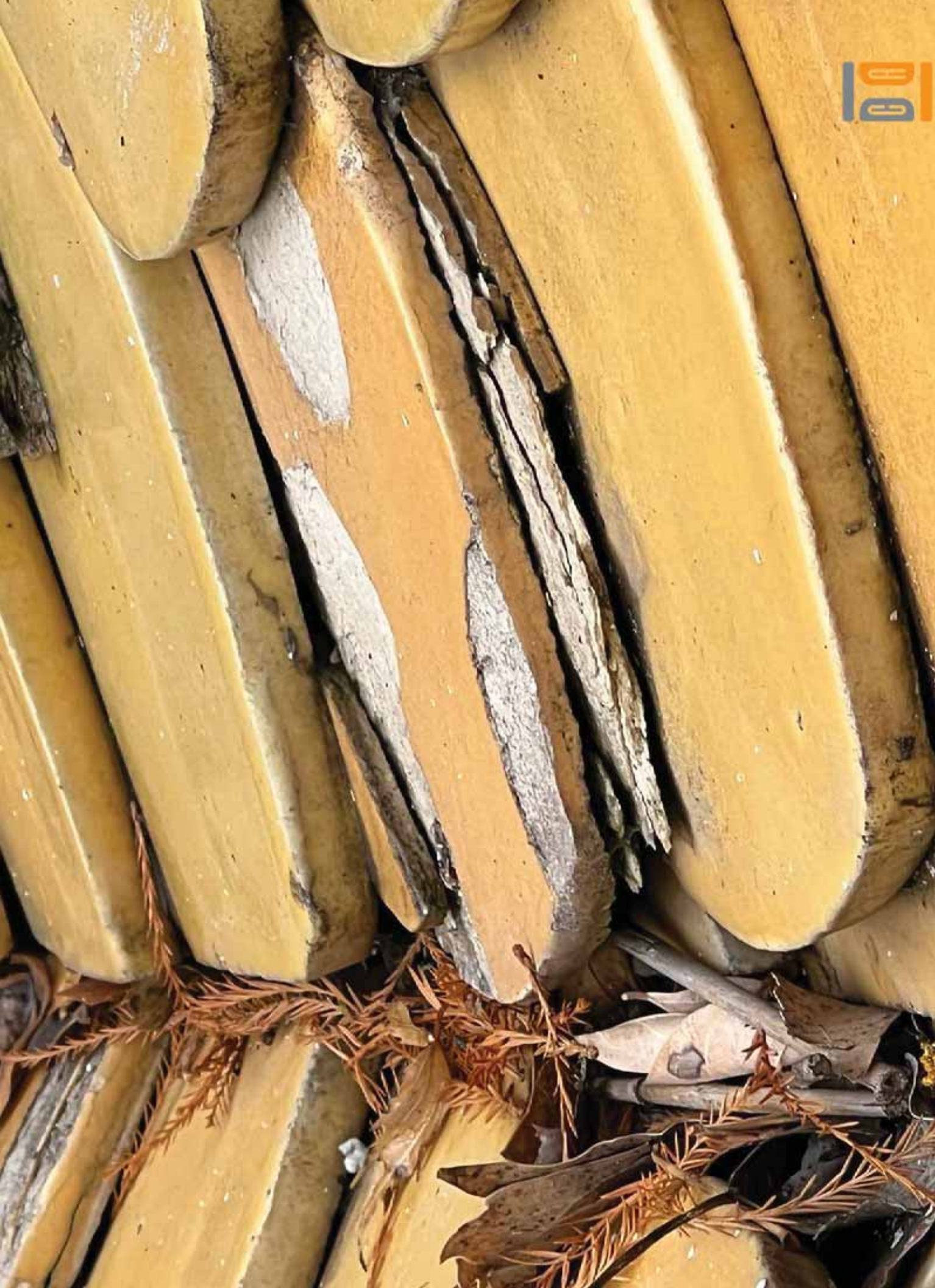
19. Close up of tile degradation at valley identified in images - Priority 1
