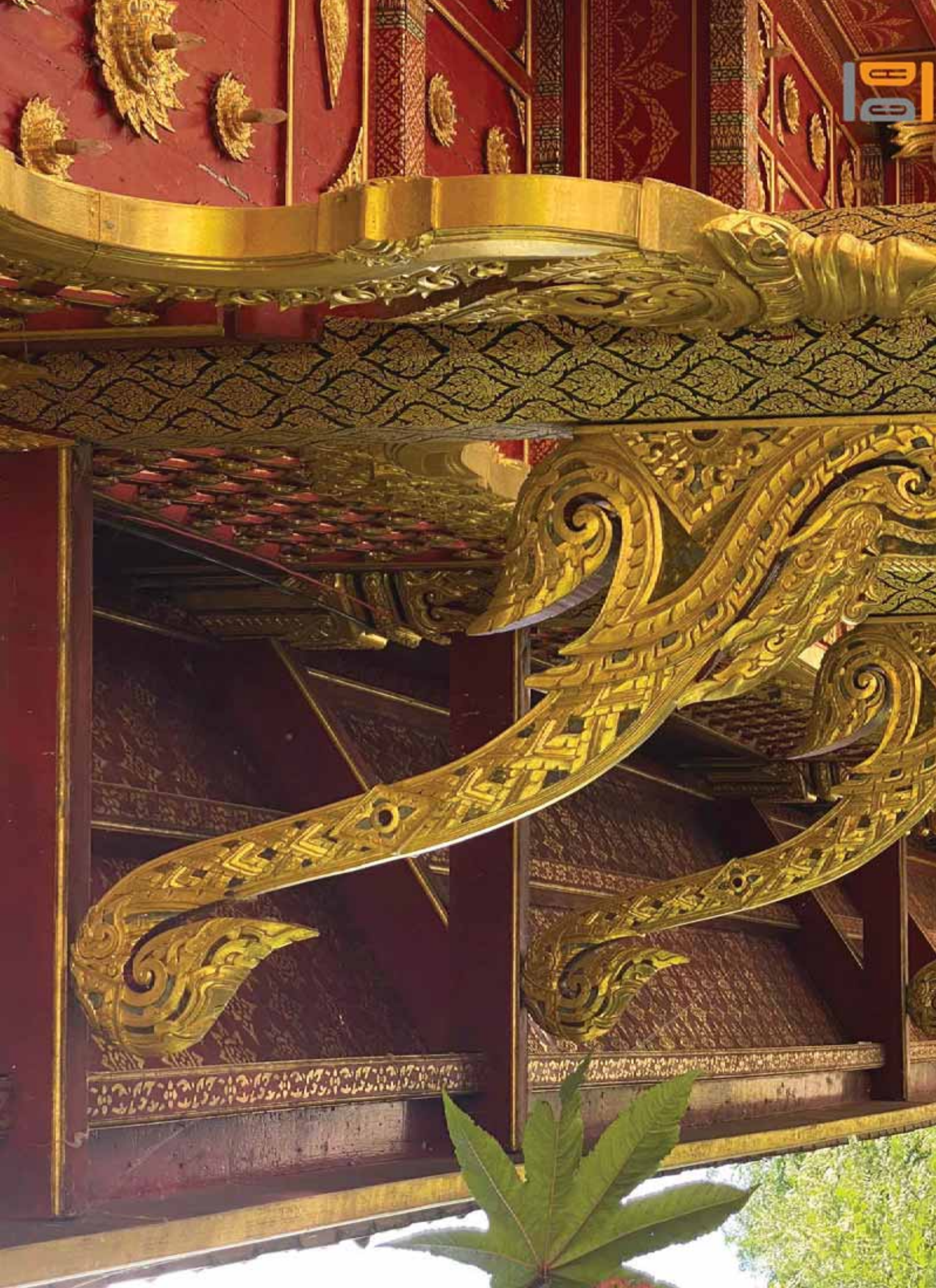
49. Exterior Condition of column capital - Priority 3
