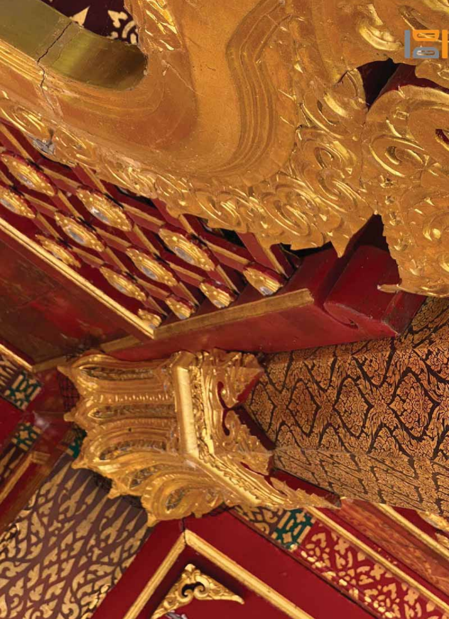
47. Interior Condition of column capital - Priority 2
