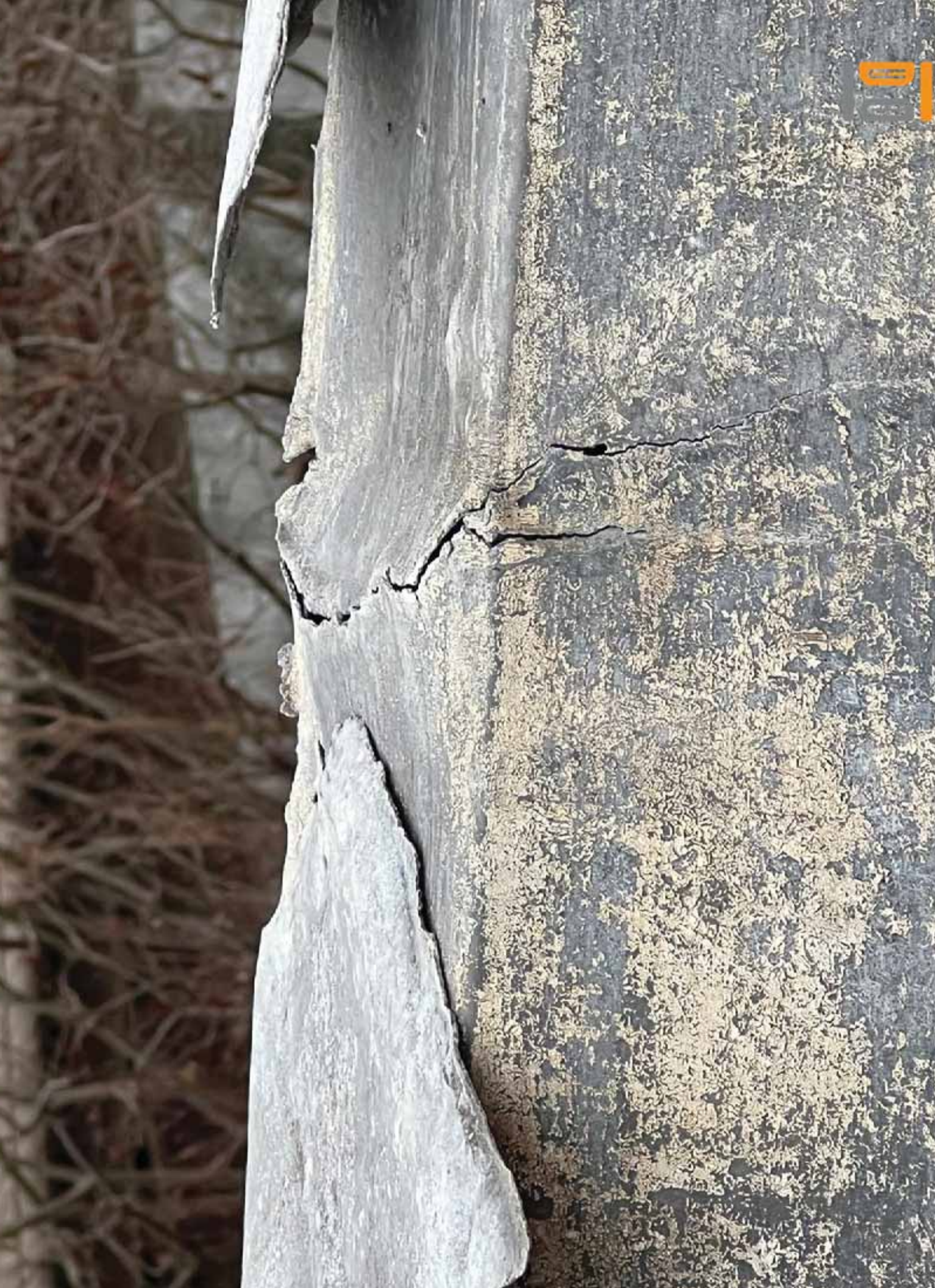
32. Degraded and fractured lead fasteners failure has led to cyclic fatigue and critical failure - Priority 1
