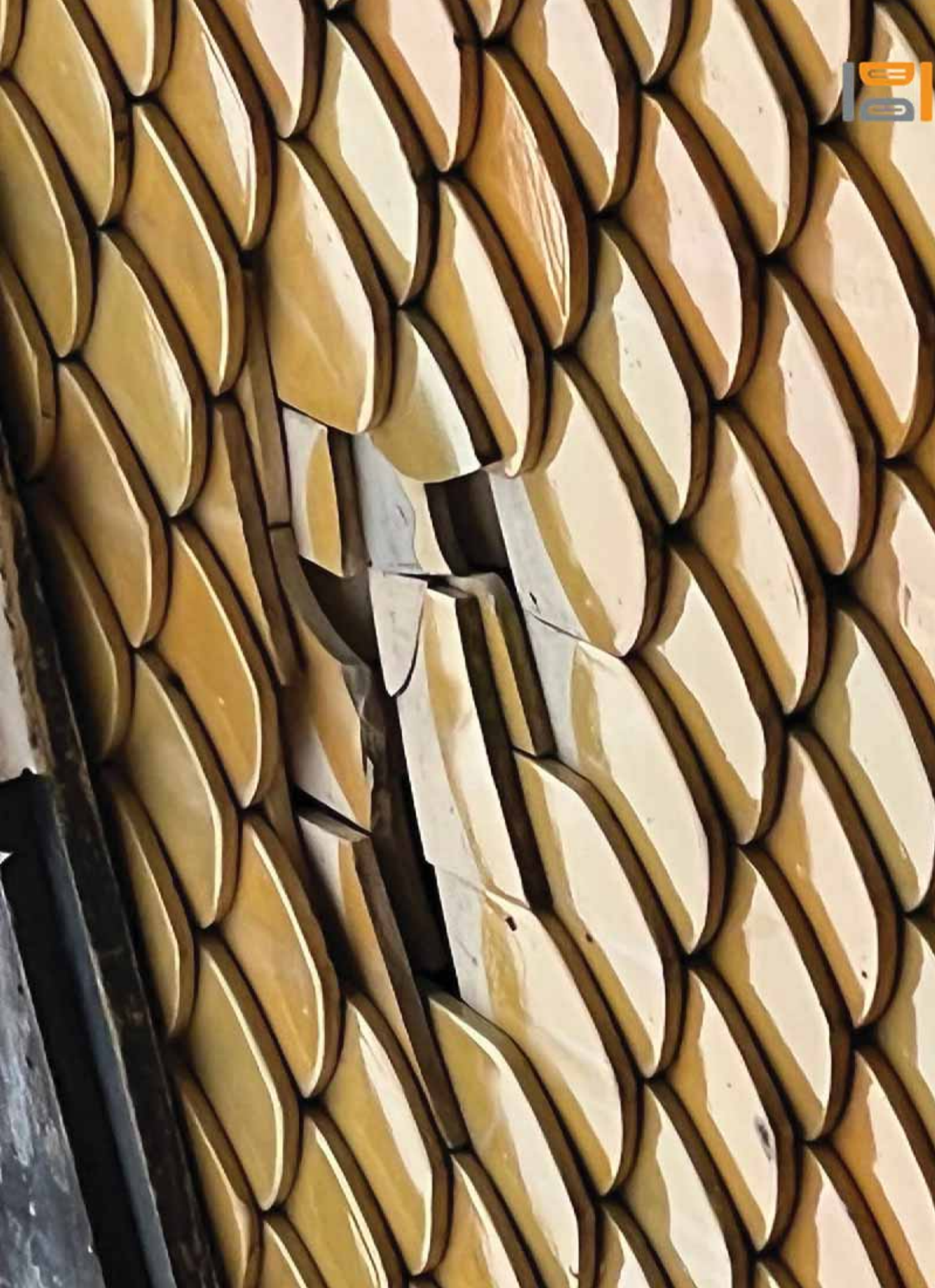
14. View of fractured tile – from impact or concentrated point load (assumed) - Priority 1
