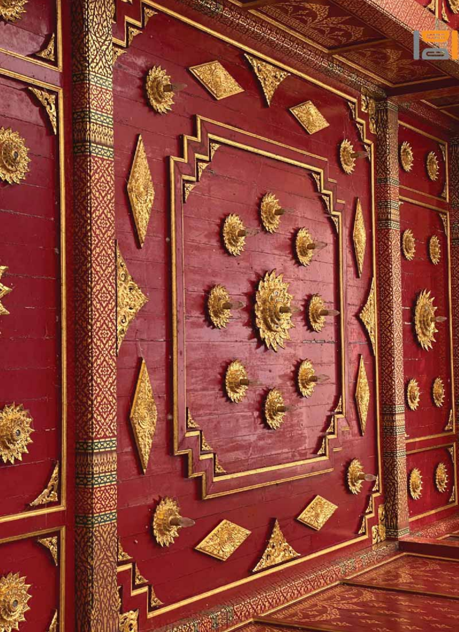
44. Interior Ceiling condition with buckling edges and paint failure - Priority 2
