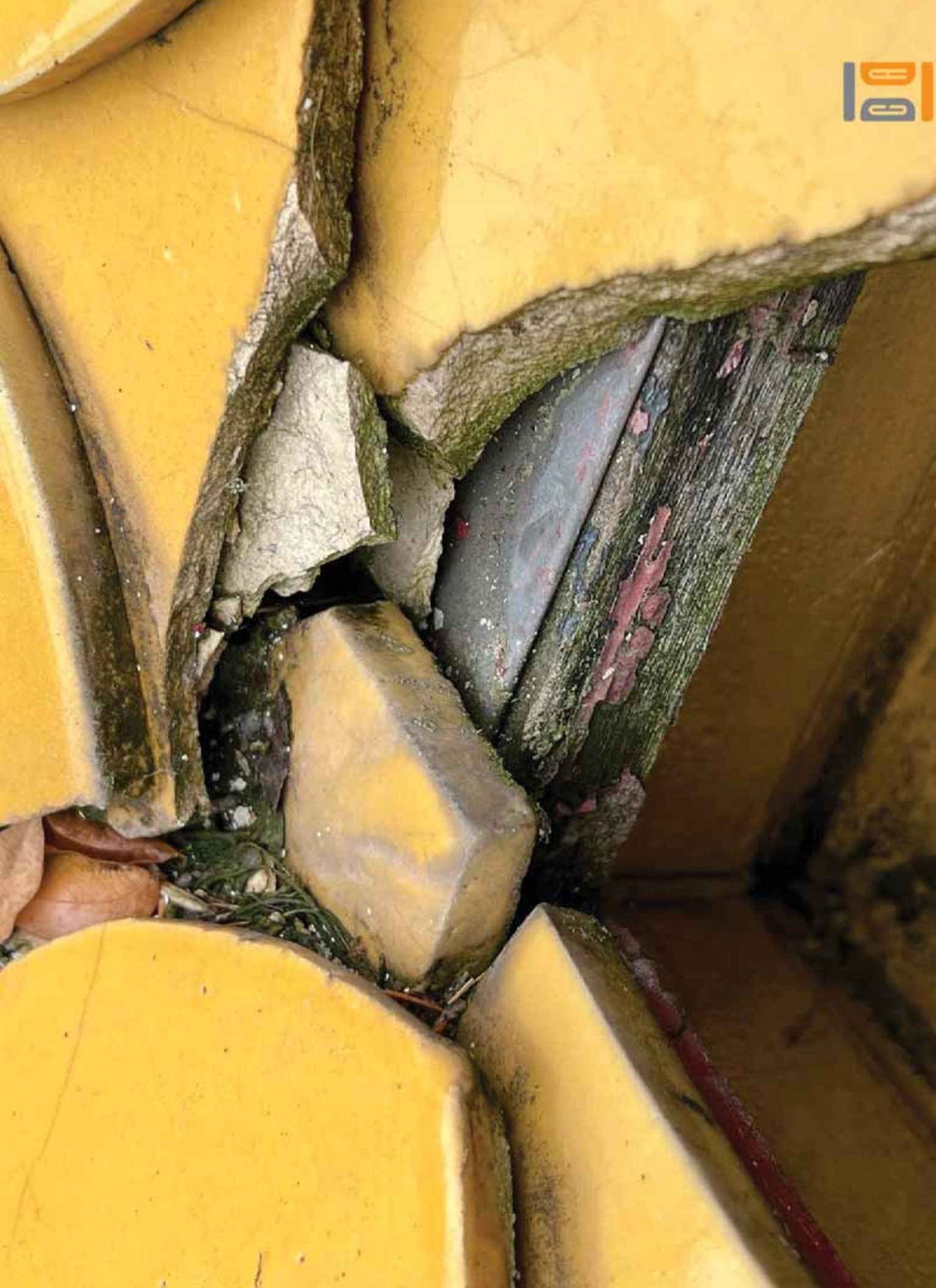
20. Close-up of valley termination at location referenced in images - Priority 1
