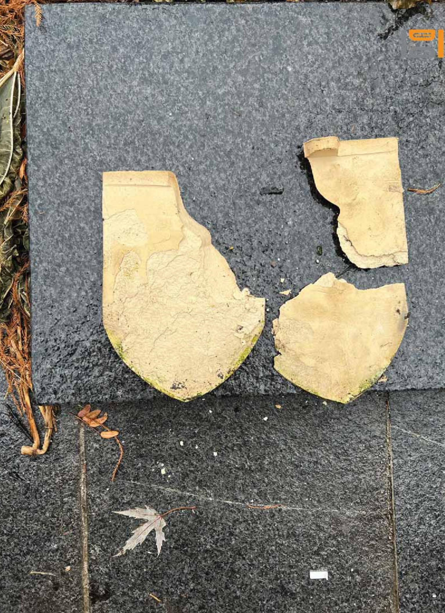
8. Exploded tile - Typical condition of water-infiltration damage - Priority 1
