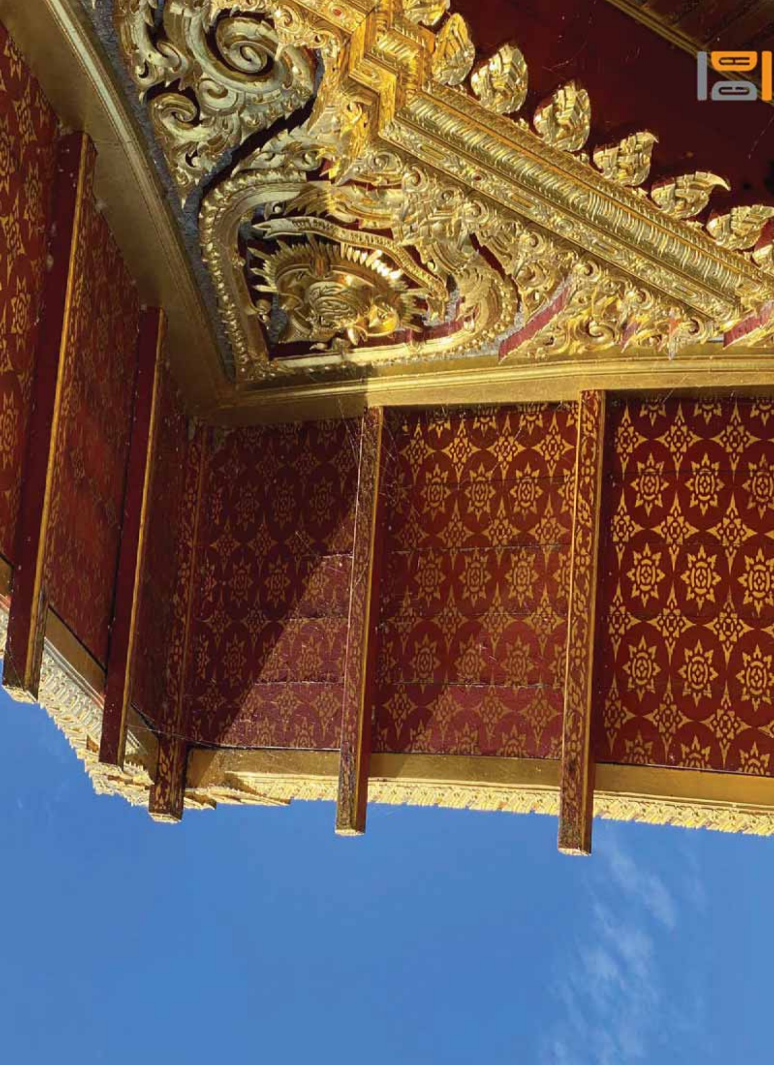
43. Roof Soffit condition with buckling edges and paint failure - Priority 2
