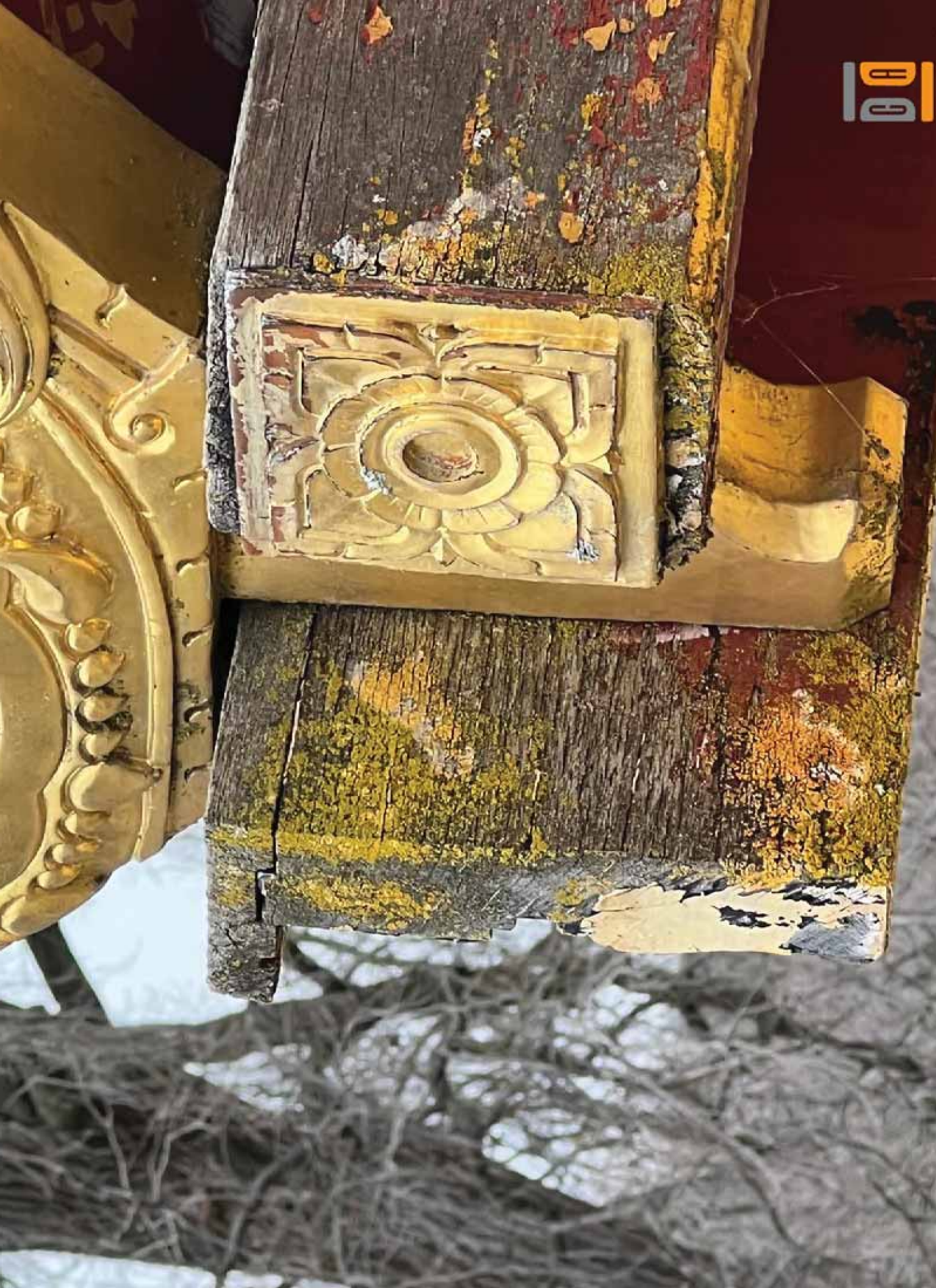
41. Repair attempts at base of hip ridge - Priority 2
