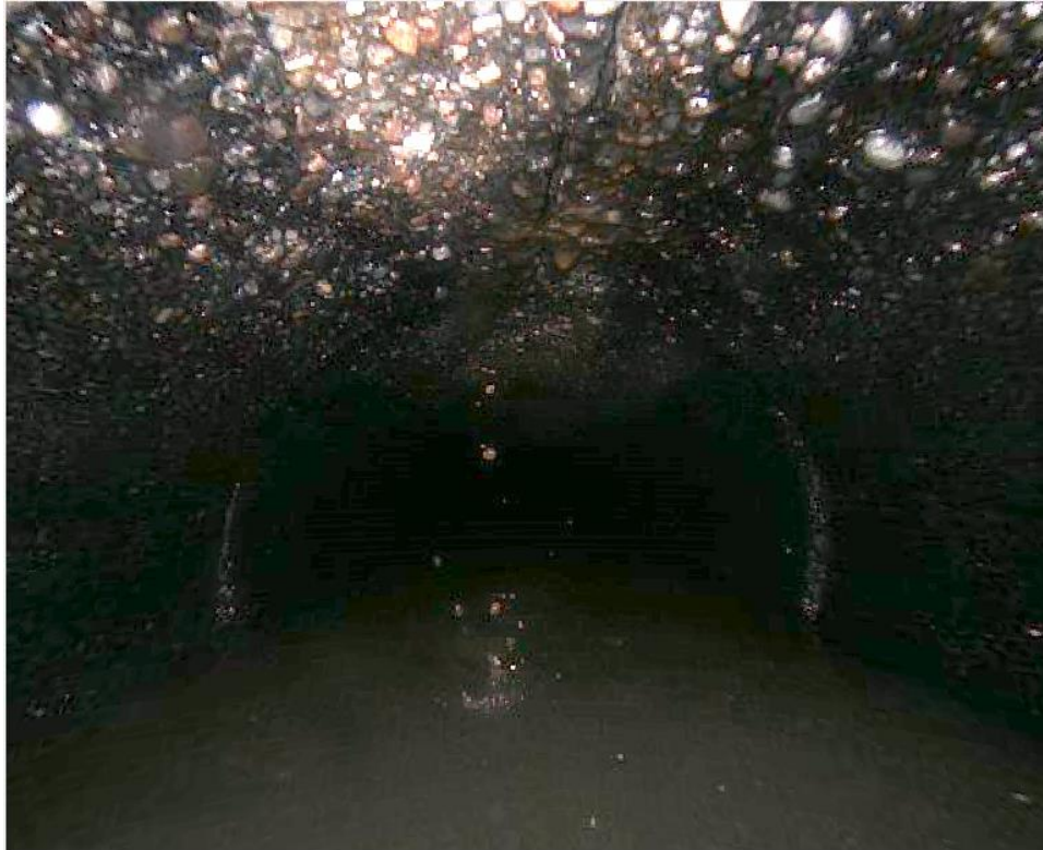
Fractures & Exposed Aggregate – Structural damage to pipe.
