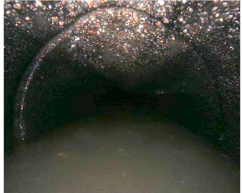
High Water Levels – Water marks indicate pipe capacity nearly full
