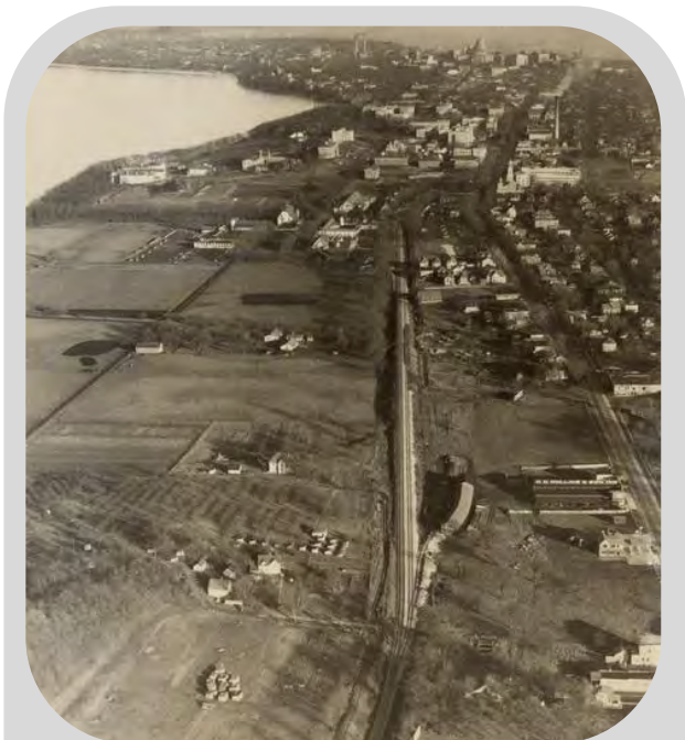
Aerial view of Isthmus looking west towards State Capitol Building in 1930. Wisconsin State Historical Society image 31351
