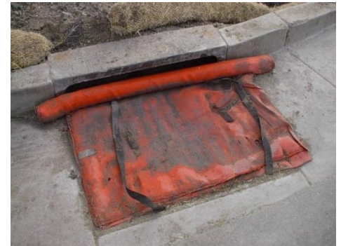
Inlet protection prevents sediment from entering the storm sewer system.
