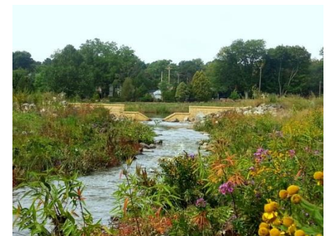
Restored Stream Channel downstream of Manitou Pond
