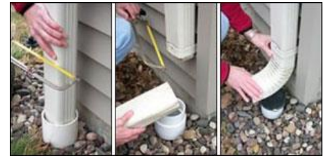
Disconnecting downspouts is an easy process. Forty percent of the homes in the watershed (1,617 homes) would be disconnected. This would entail rerouting 25% of a home's roof area to a turf area (i.e., 1 of 4 downspouts), rather than a paved area.
