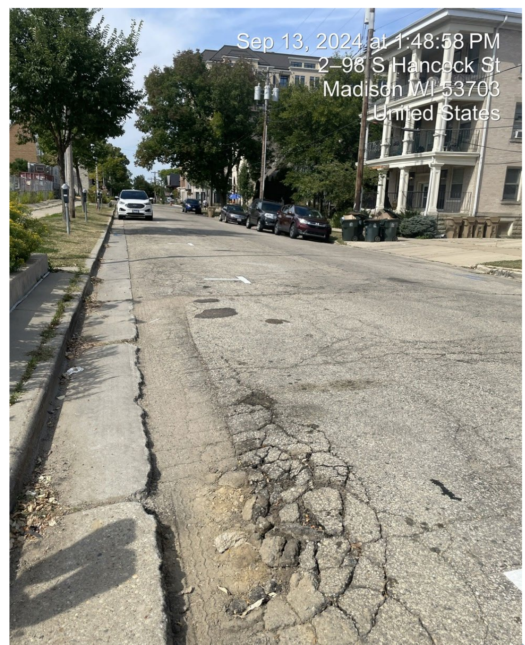
In front of southern rain garden, looking north towards East Wash
