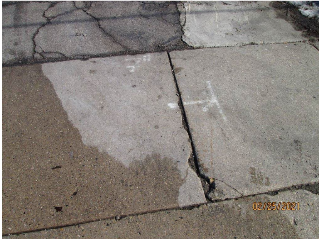
Voids and Erosion of Joints
