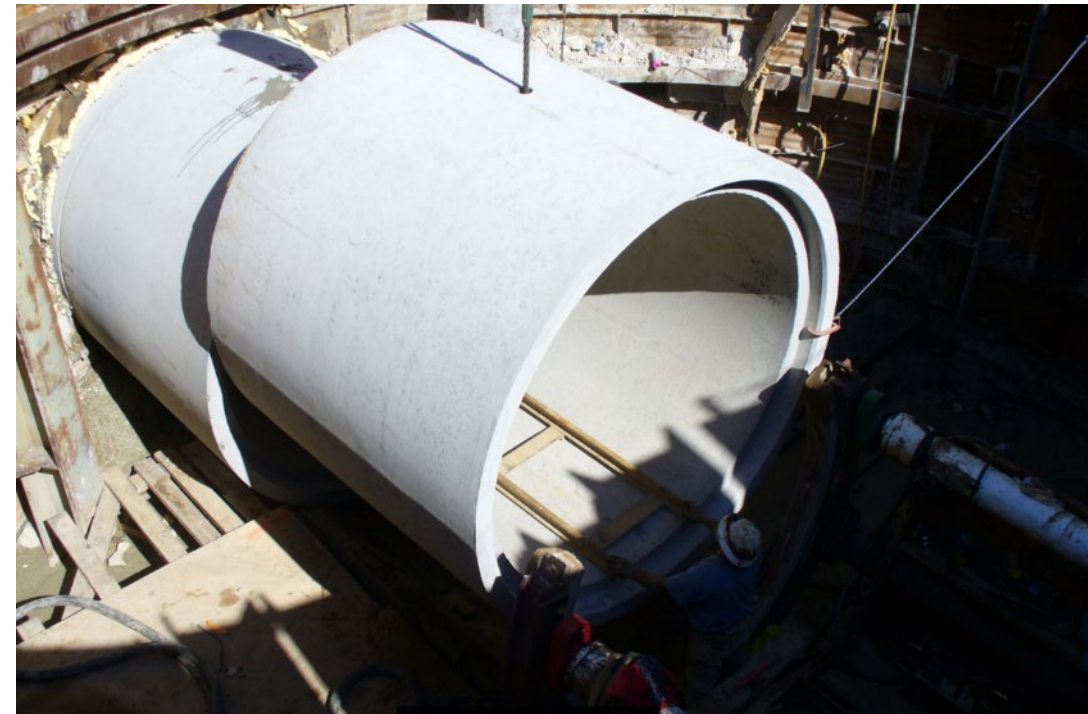
96" pipe tunneling on University Ave, Madison, WI (2013)
