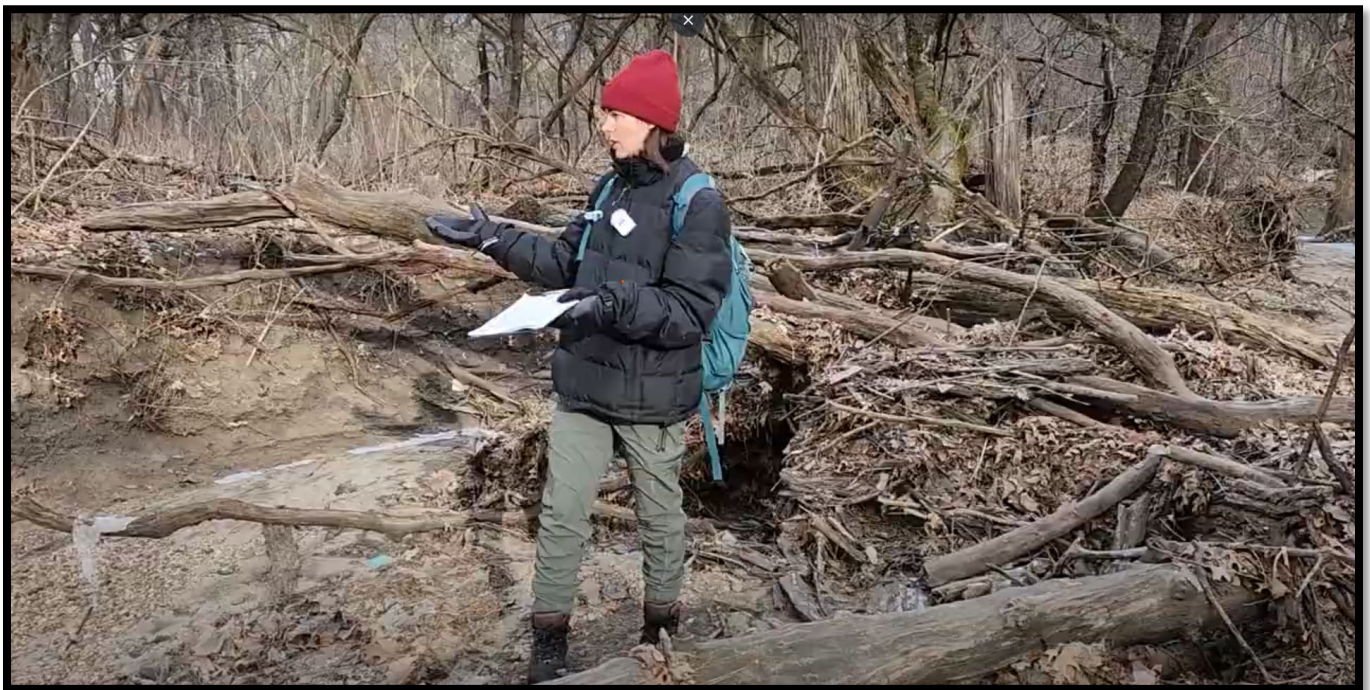
Figure 4 Log dam created a channel blockage and led to erosion on adjacent bank
