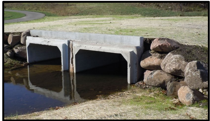
Figure 62 – Example of a box culvert
