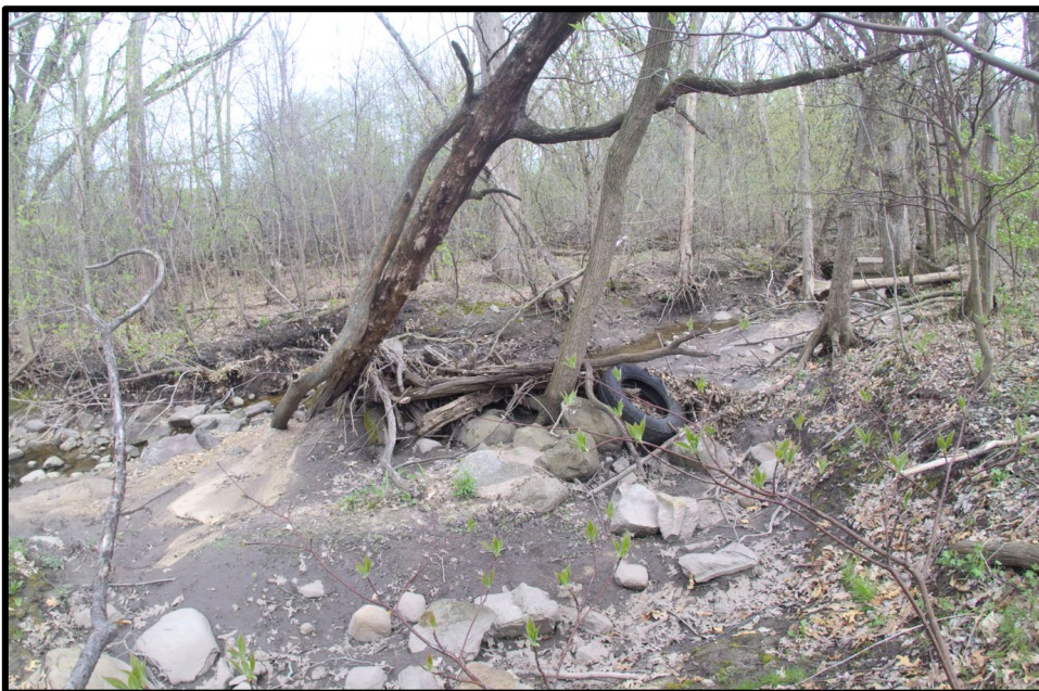
Figure 7 Channel widened due to erosion. Can see widened channel section in foreground near tire.
