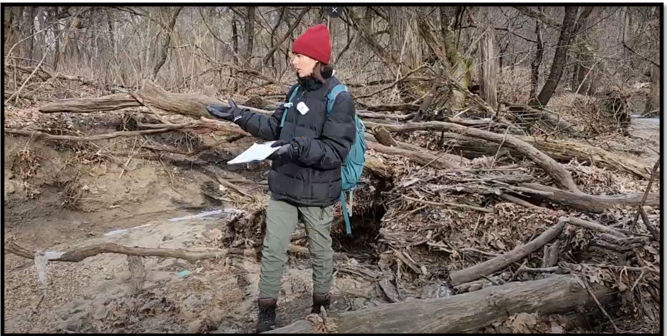
Figure 4 Log dam created a channel blockage and led to erosion on adjacent bank
