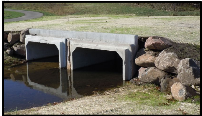
Figure 62 – Example of a box culvert
