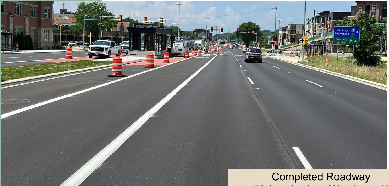
Completed Roadway (University Ave. Eastbound.)
