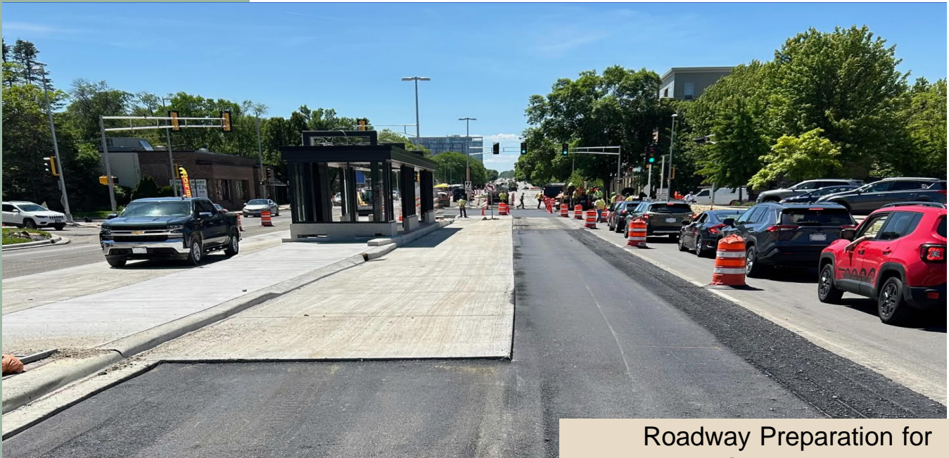
Roadway Preparation for Asphalt Surface Installation
