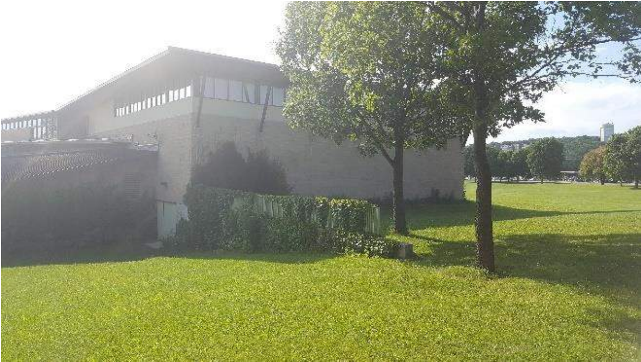
Figure 8: East wall of gymnasium.
