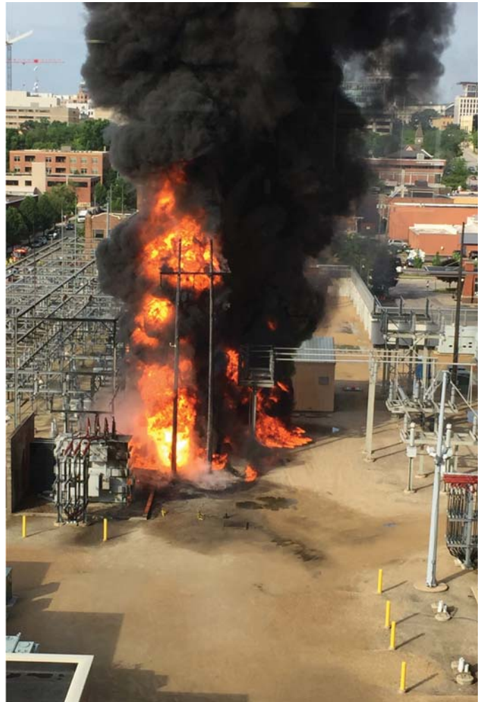
Photo from the July 19, 2019 transformer fire at MG&E
