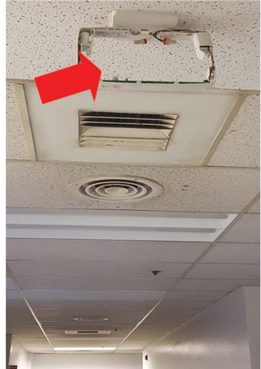
The arrow is pointing to a missing exit sign, which is a fire code violation.
