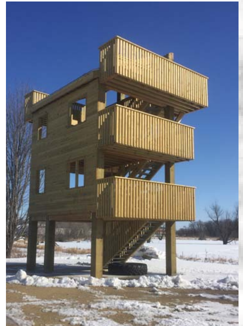
Newly-built Ladder Training Tower at Station 14 on Dairy Dr.
