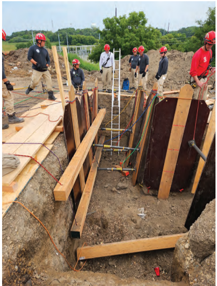
Above: In August, HURT members trained with Fitchburg Fire Department for a refresher training on trench rescue.
