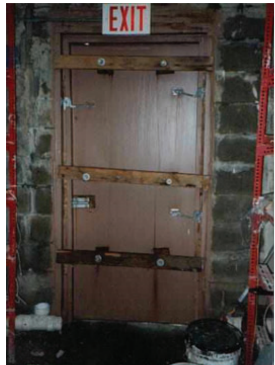
An obstructed exit is one of the most common fire code violations--and a potentially dangerous and deadly one.
