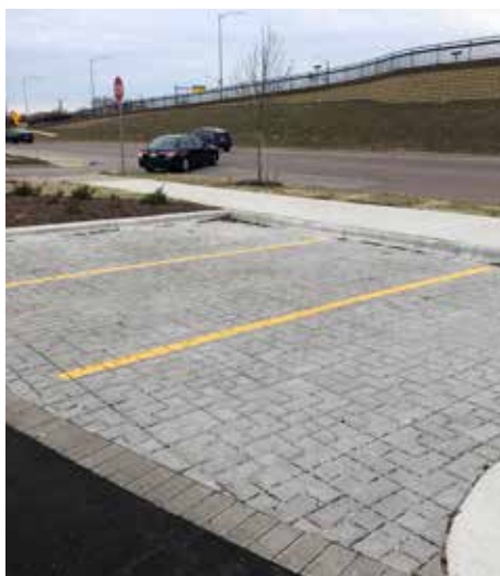
Pervious pavement at Portillos at West Towne.
