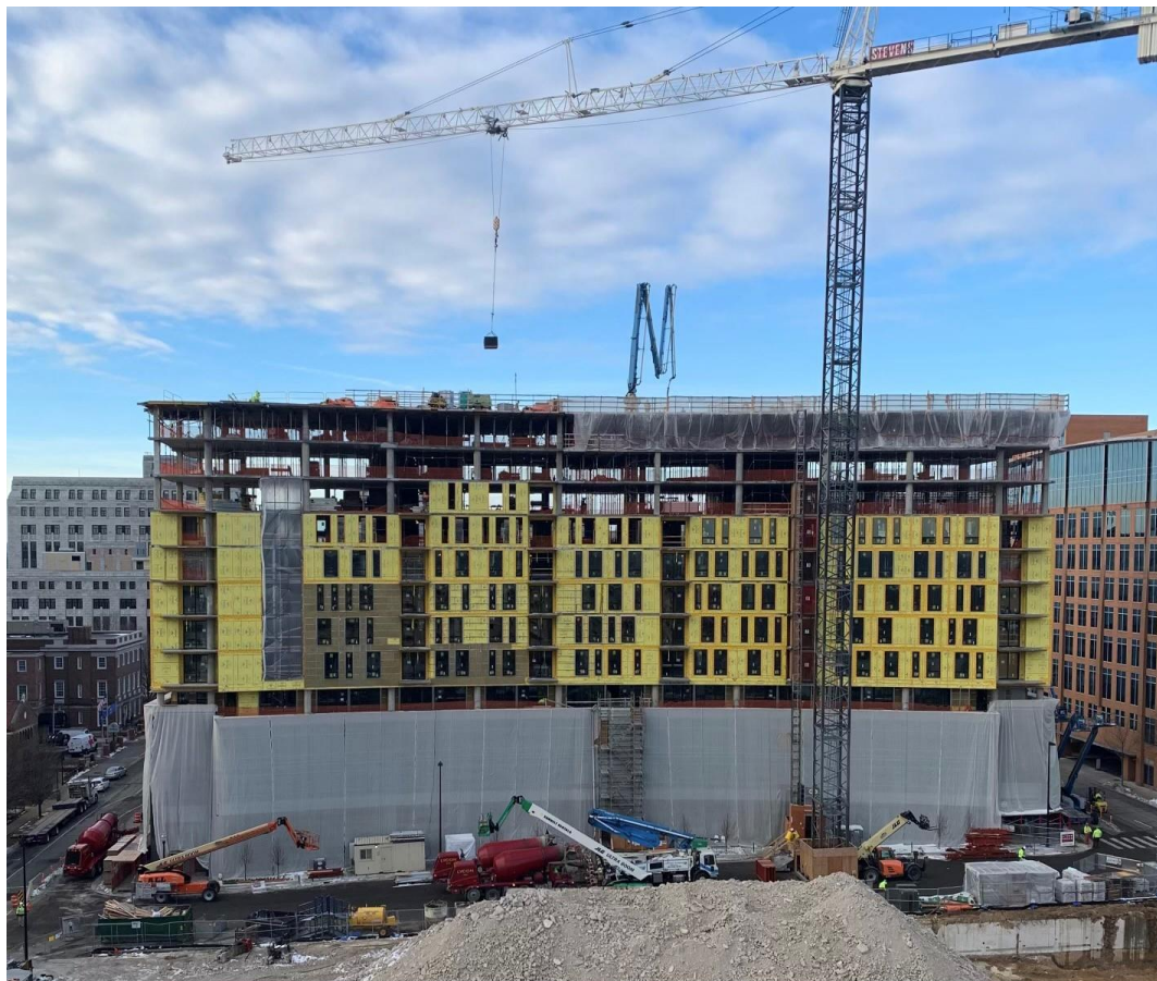
Stone House apartment construction progress on Block 88 looking west
