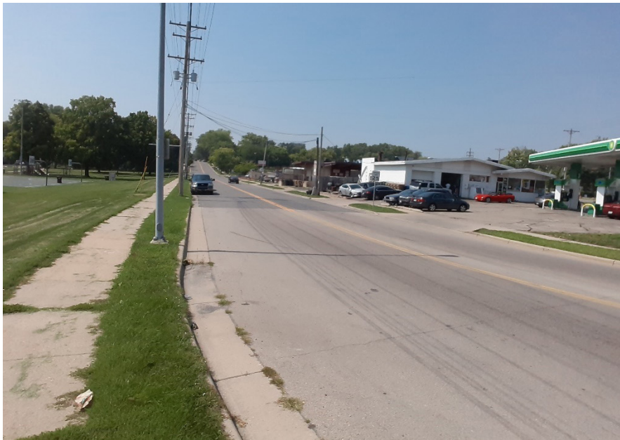
Figure 7. It is likely that crossing improvements will be a component of the Project, as many roads such as Troy Drive currently lack low-stress bike facilities.
