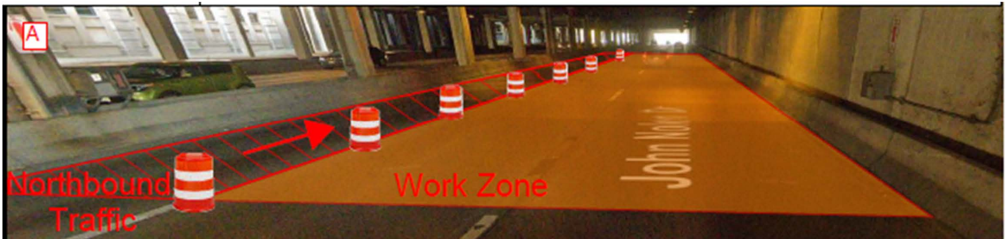
Example Traffic Control Lane Closures
