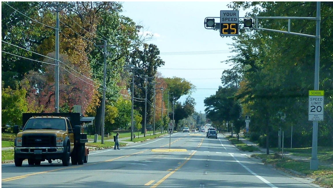
Image 1. Pedestrian island with TWLTL at Farragut Street, looking south.
