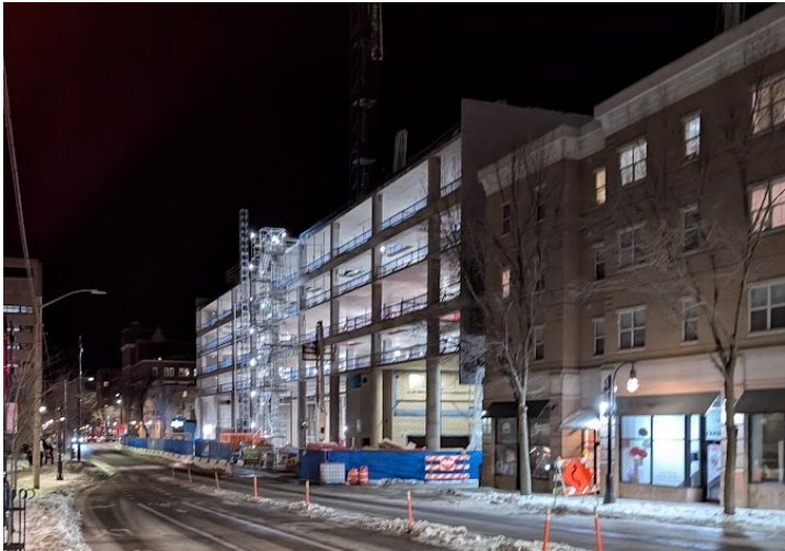
Figure 18 Lake St Garage
