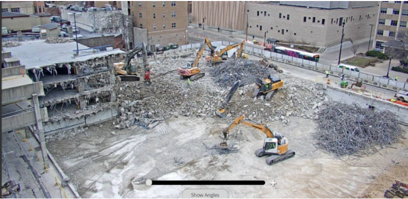
Figure 35 Demolition of State St Campus Garage Began in January 2024
